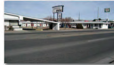
Multiple Curb Cuts
