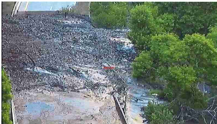
Debris flow covering eastbound lanes of I-70 4
