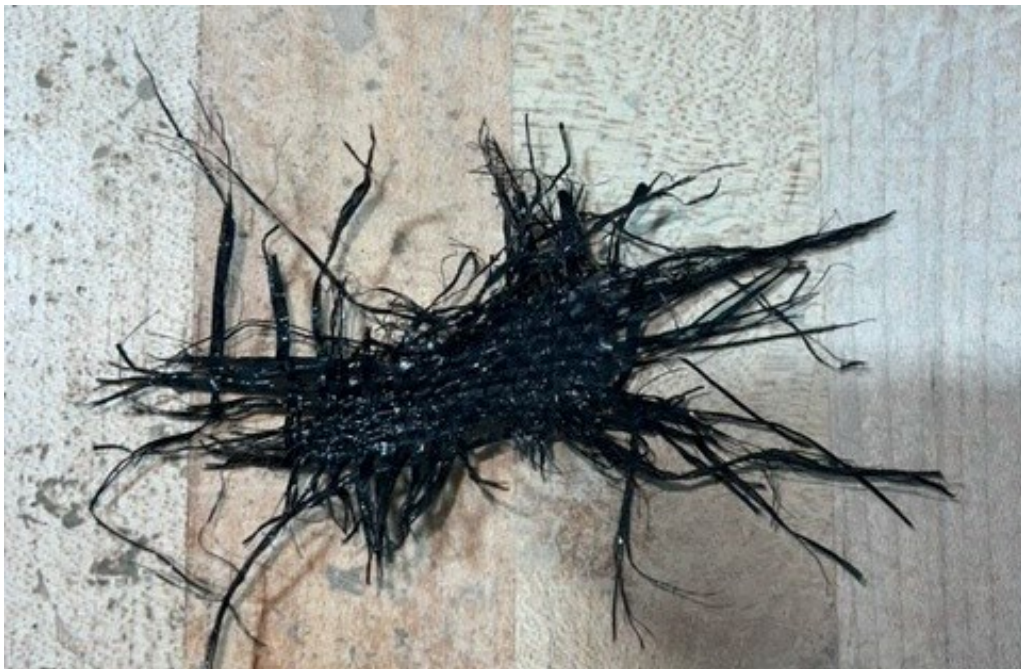
Figure 4 – Woven Geotextile Encountered below HMA in Borehole BH-3
