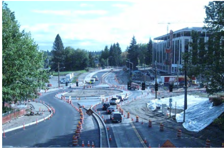
(Photo courtesy of WSDOT)
