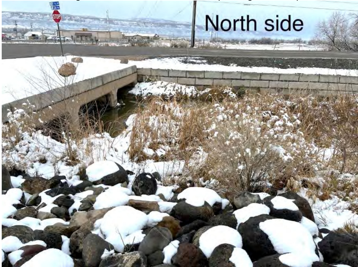
Image 4 – North Side of F 1/2 Road CBC (Looking southwest)
