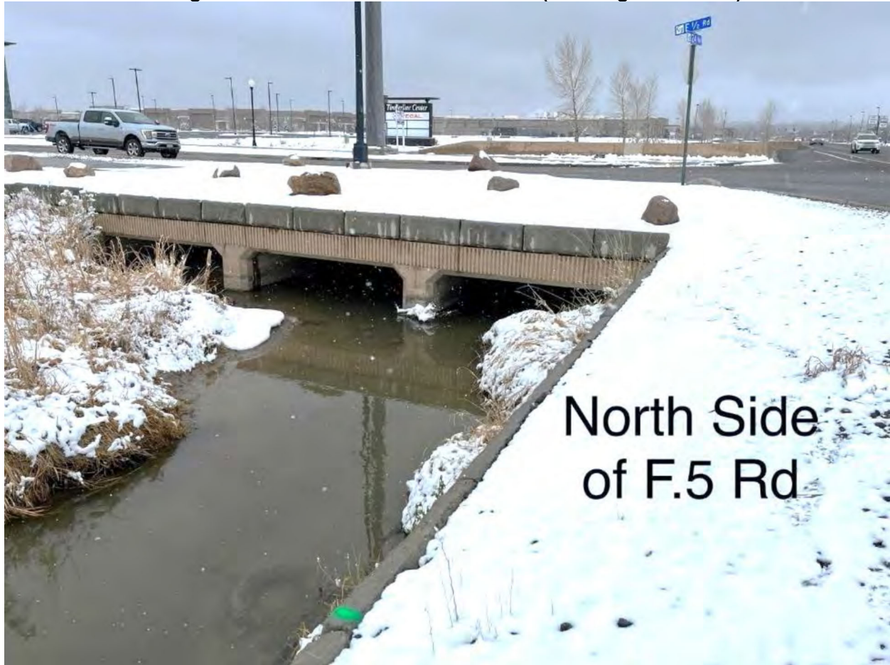
Image 3 – North Side of F 1/2 Road CBC (Looking Southeast)
