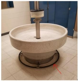
**Answer**: The metal bar around the bottom of the sink will be removed but the brackets that hold the bar will not be removed.
