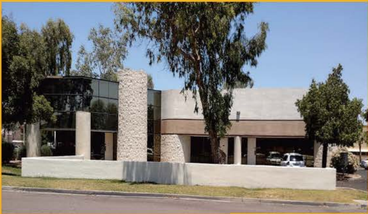
Disaster Recovery Facility Tempe, Arizona
