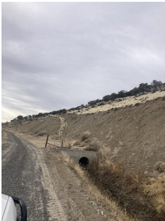
Figure 4: Ditch enters ~1200LF of corrugated metal pipe along steep hillside prone to instability; gaining infrastructure in need of replacement
