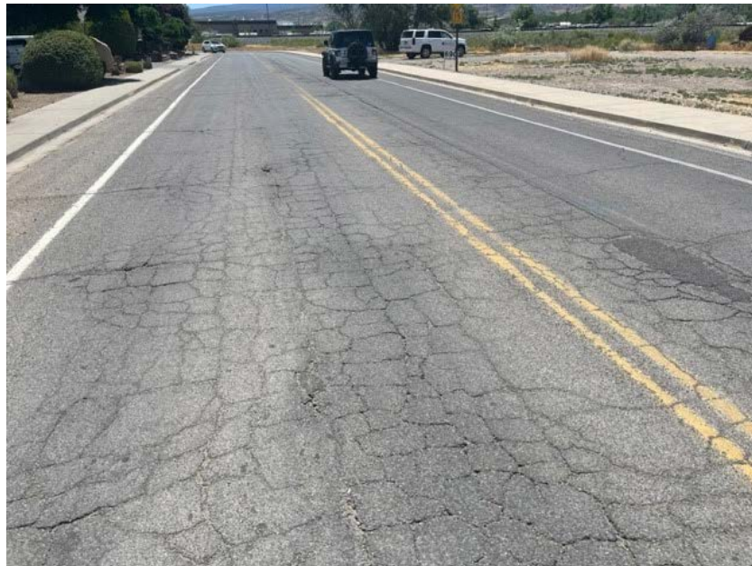
Figure 4 – Severe Fatigue Cracking Distress on Crosby Avenue
