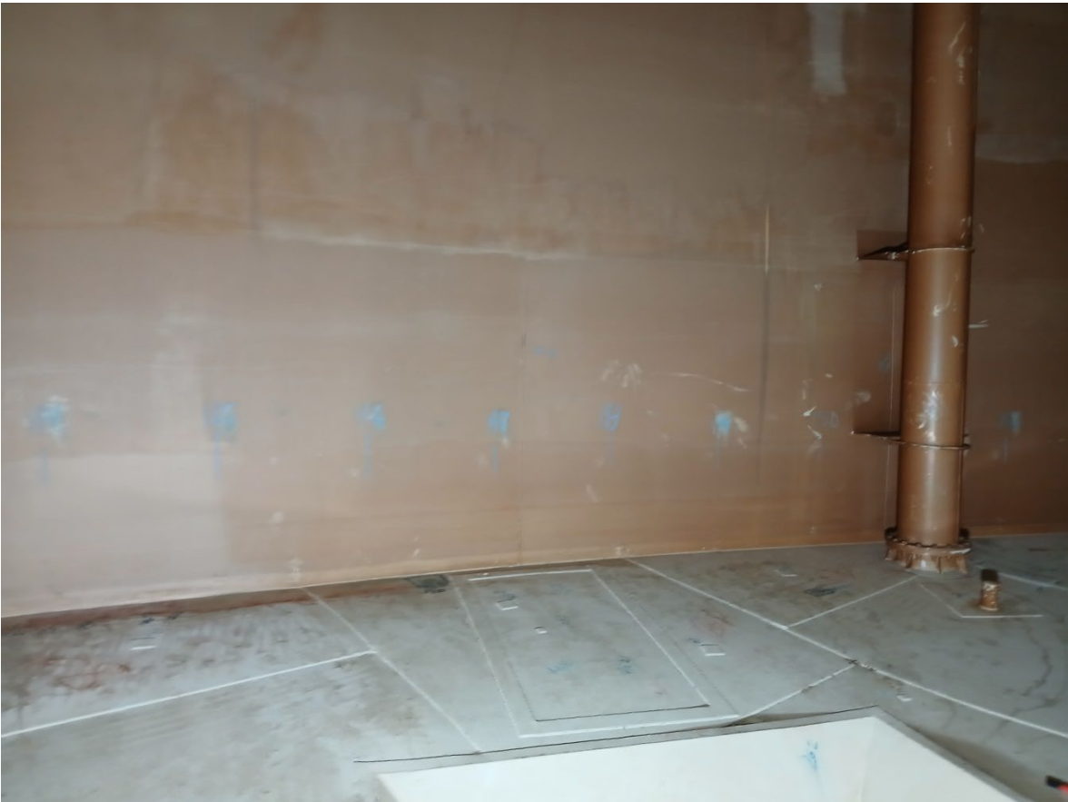
Photo 40. Patch plates around the sump
