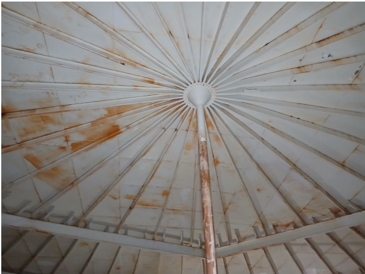
Photo 50. Underside view of roof at center column
