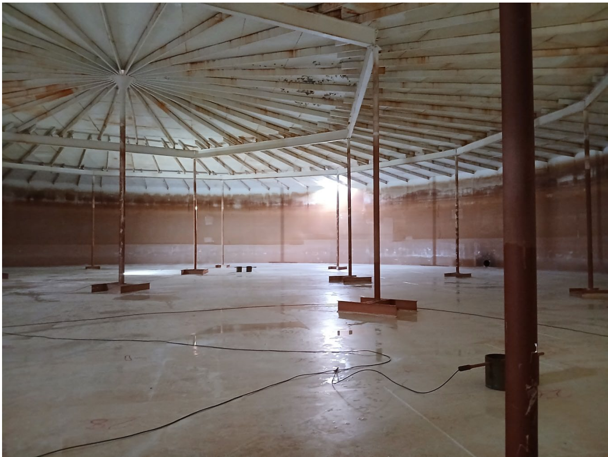
Photo 25. Interior view of tank
