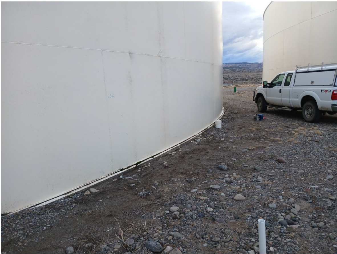
Photo 07. Tank support configuration and surrounding grade
