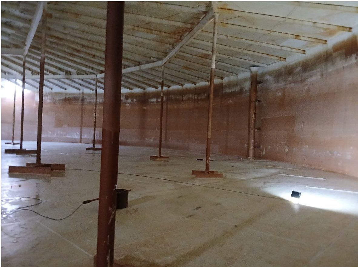
Photo 26. Interior view of tank
