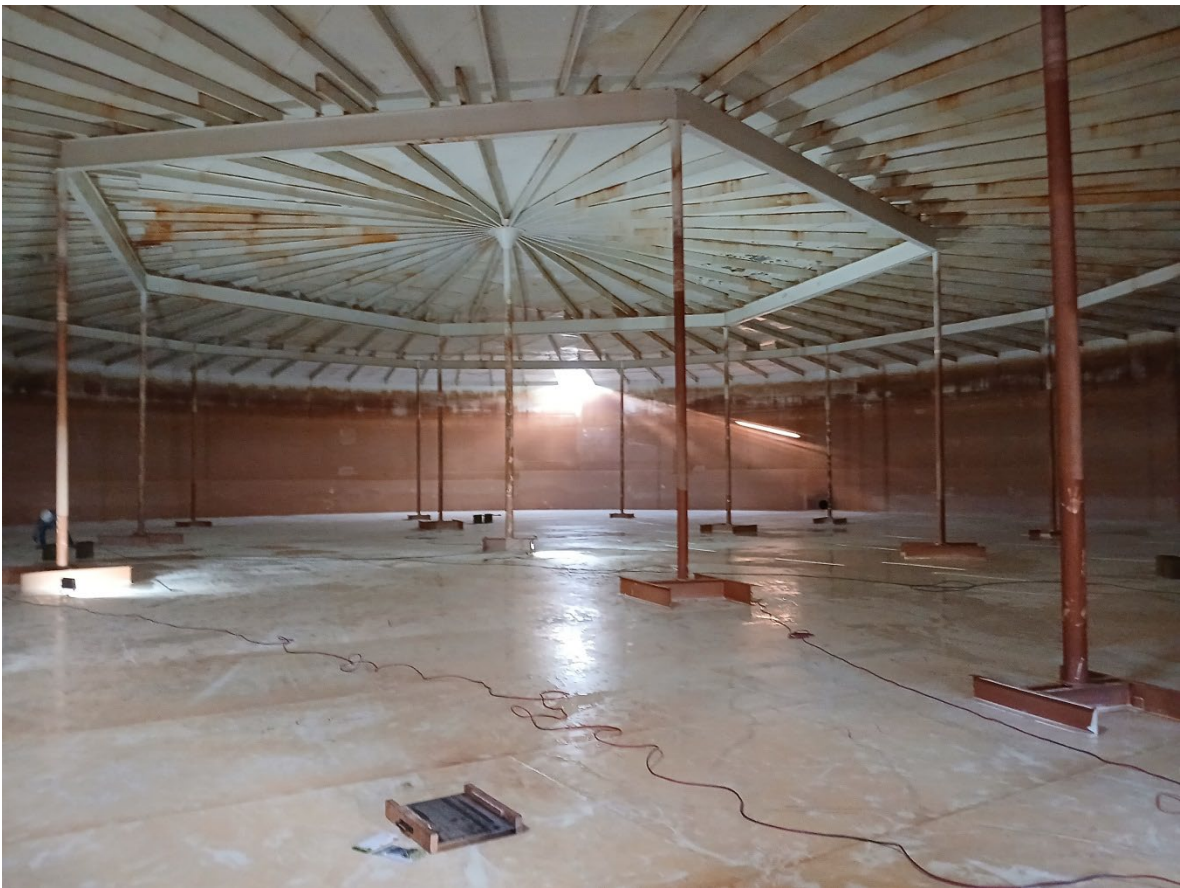
Photo 23. Interior view of tank
