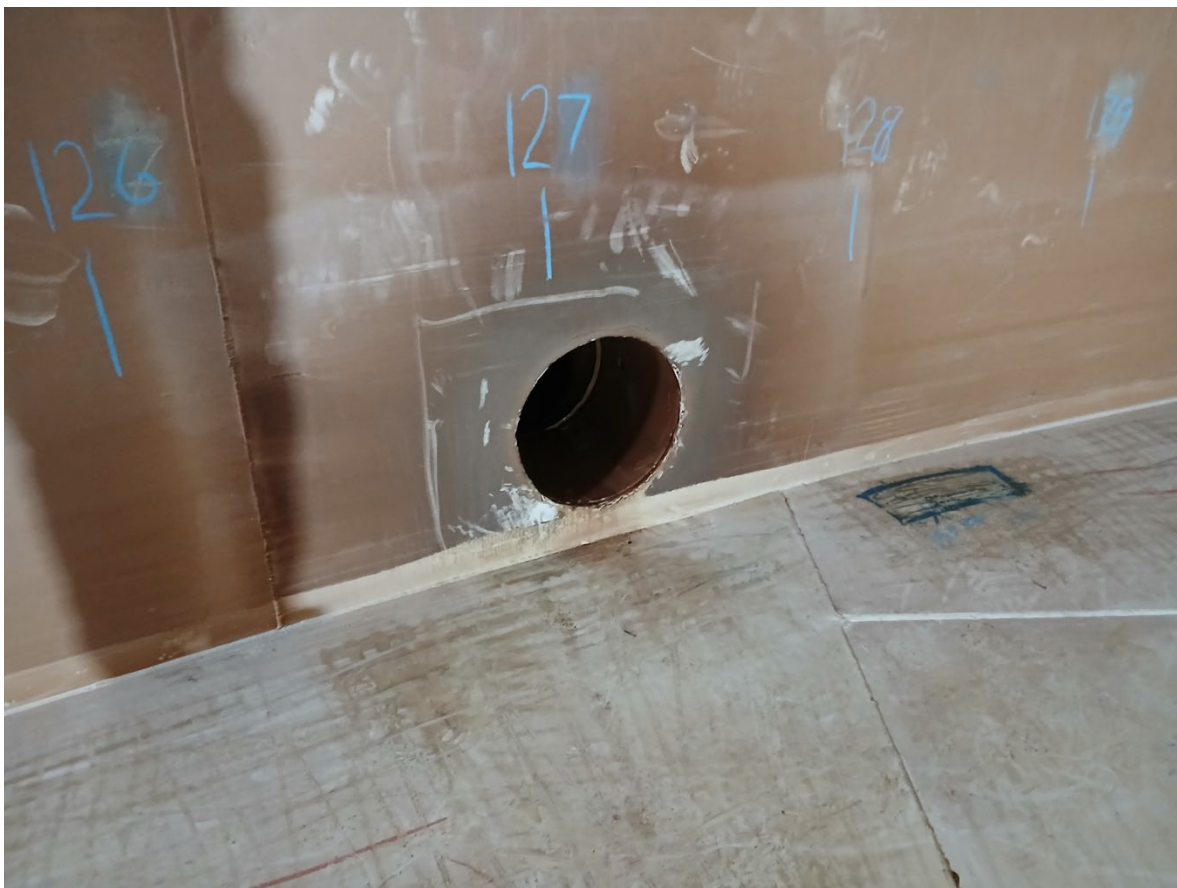
Photo 31. Interior view of shell outlet nozzle
