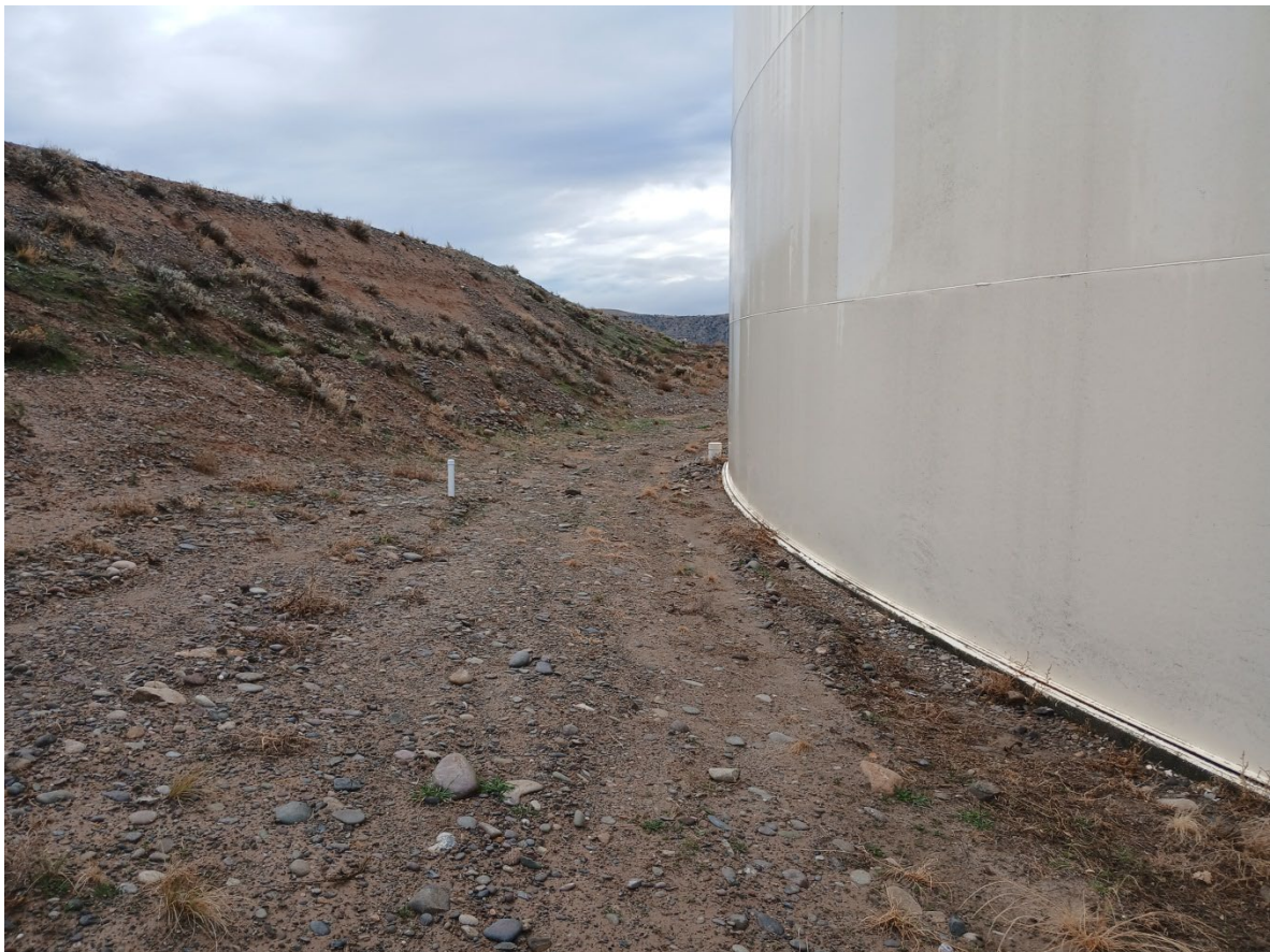
Photo 08. Tank support configuration and surrounding grade
