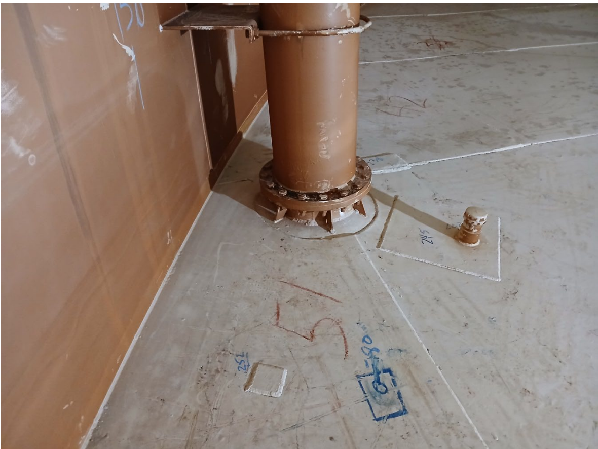
Photo 44. 16" overflow pipe
