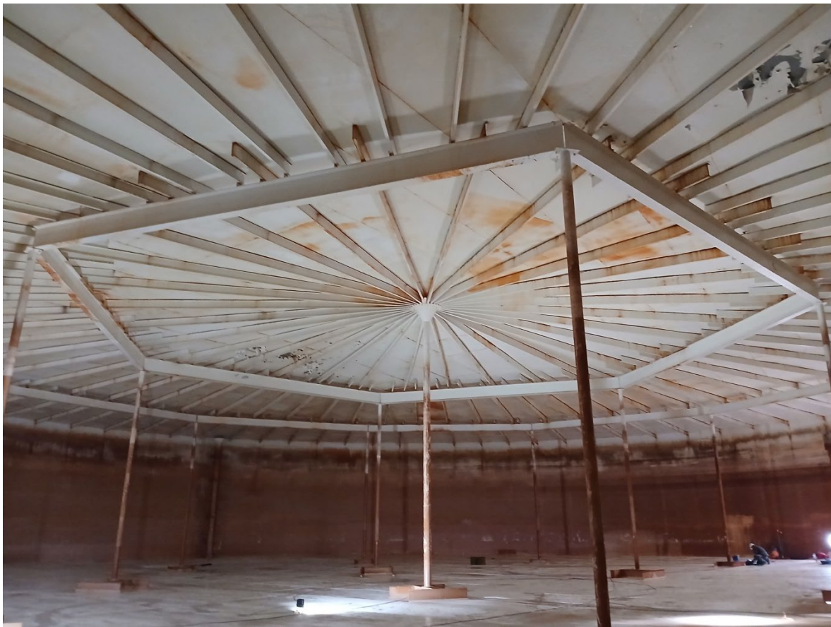
Photo 49. Underside view of roof
