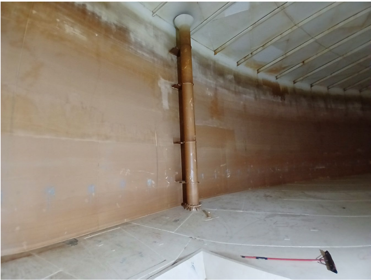
Photo 43. 16" overflow pipe
