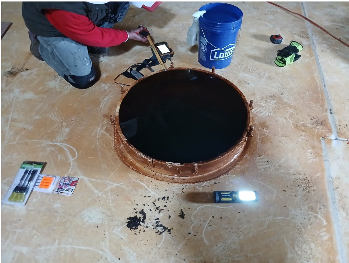
Photo 27. 30" bottom inlet pipe configuration with silt stop and water inside
