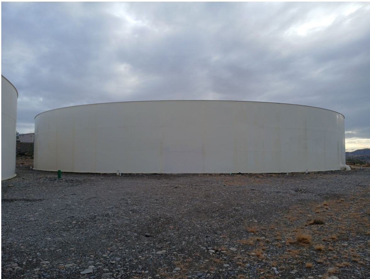
Photo 01. Grand Junction Water Treatment Plant, 4 MG, 170' Diameter Water Tank
