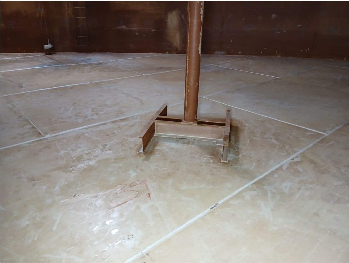
Photo 47. Roof support column and base configuration
