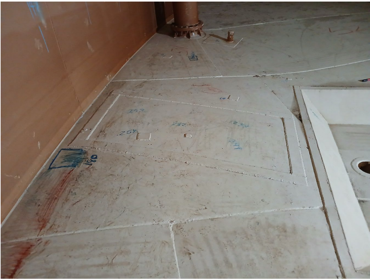
Photo 41. Patch plates around the sump
