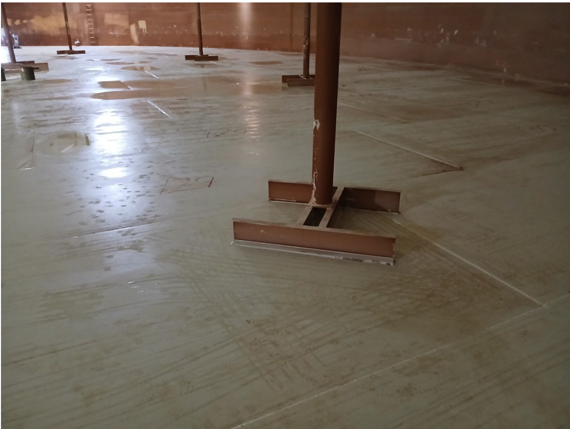
Photo 46. Roof support column and base configuration
