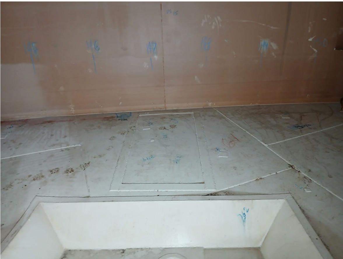
Photo 39. Patch plates around the sump
