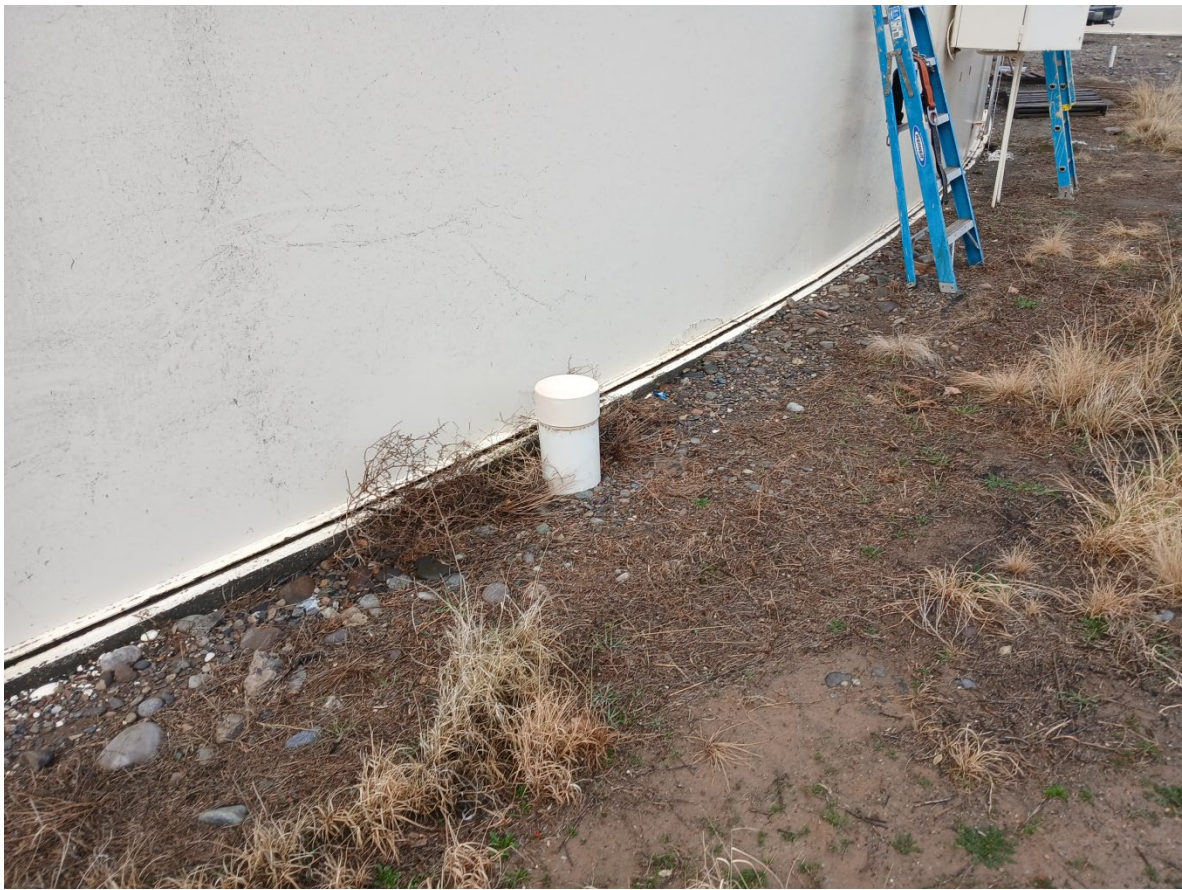
Photo 09. Tank support configuration and surrounding grade
