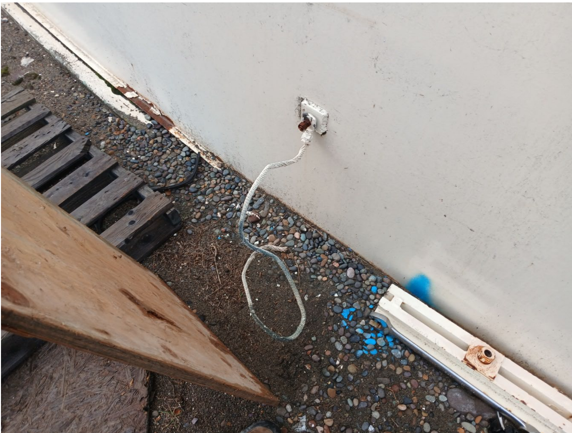
Photo 19. Two (2) of two (2) grounding wires at bottom of tank
