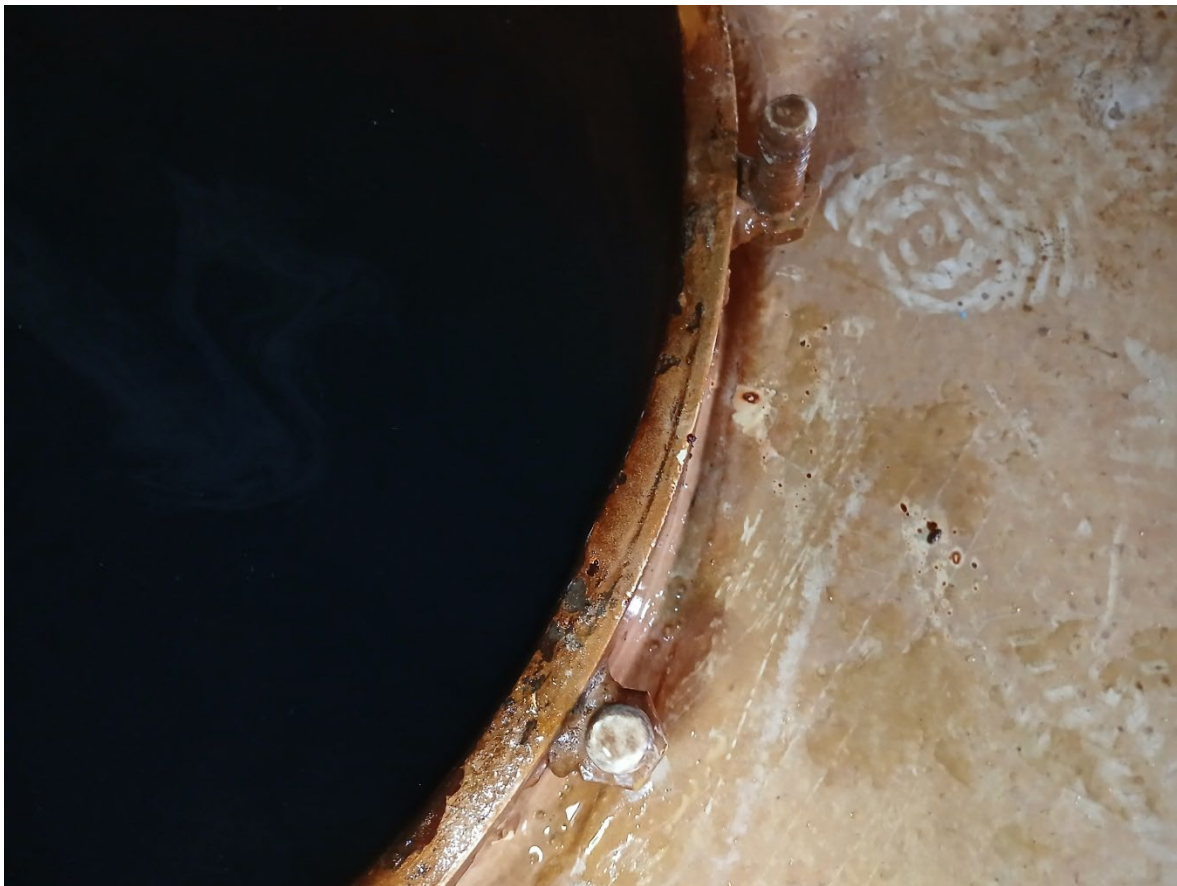
Photo 28. 30" bottom inlet pipe configuration with silt stop and water inside
