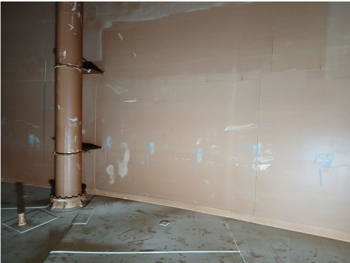
Photo 52. Two (2) of three (3) door sheets on shell
