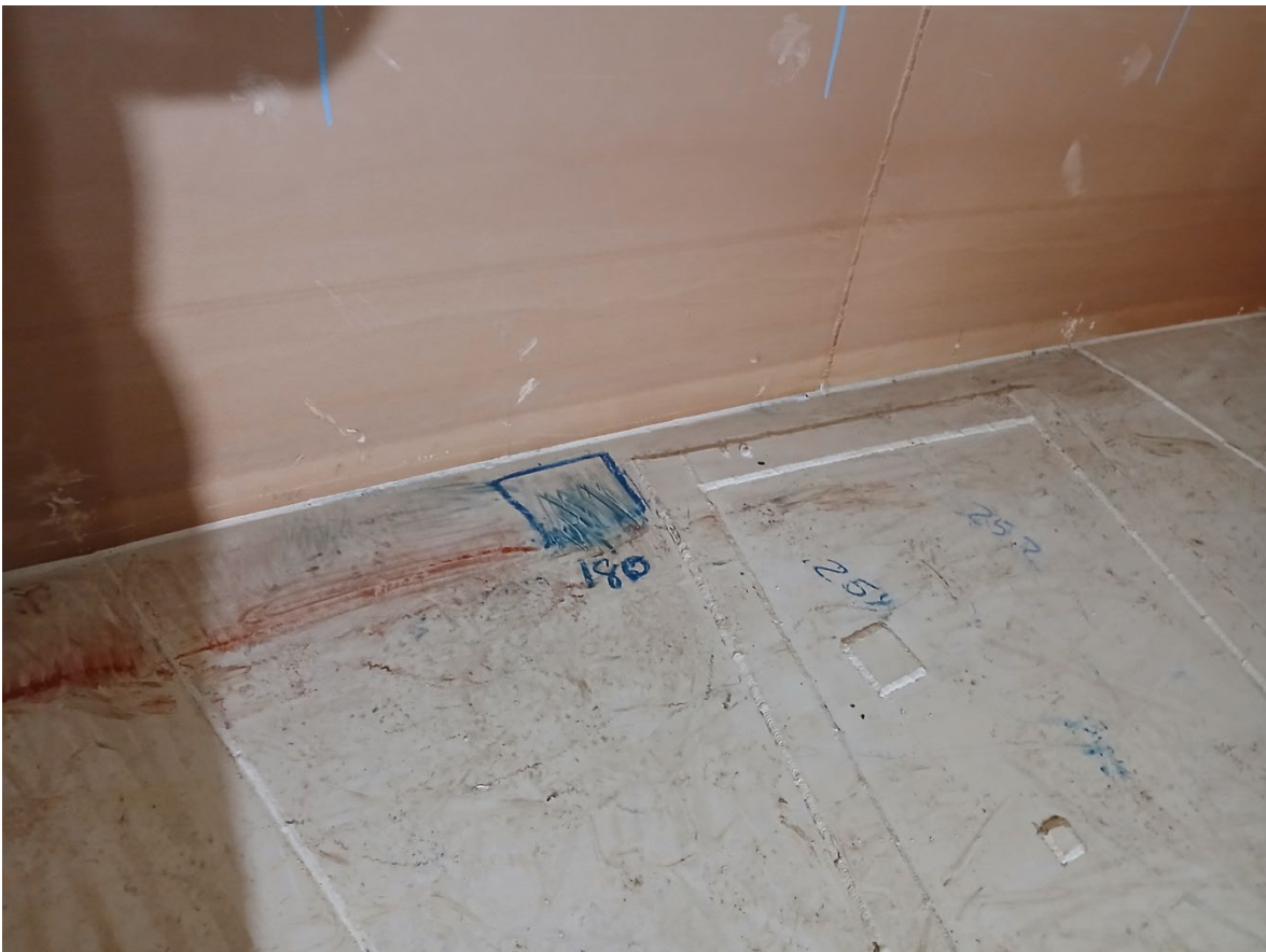
Photo 56. Example soil side corrosion / pitting at suspected edge of concrete ring wall
