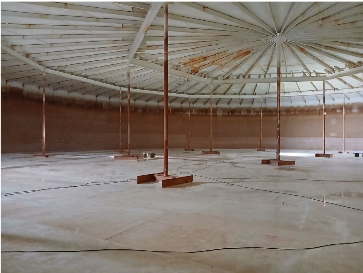
Photo 24. Interior view of tank
