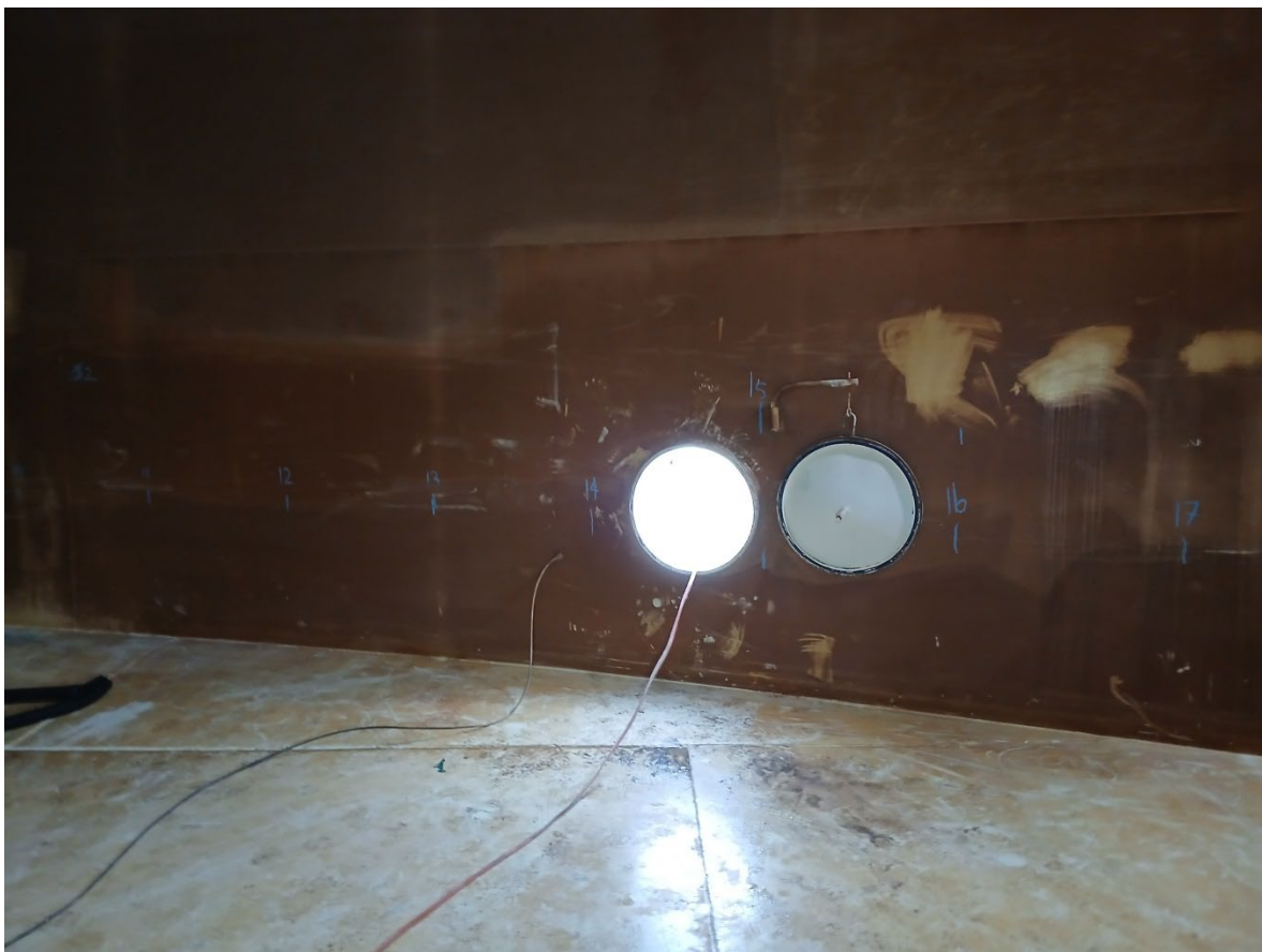
Photo 06. Interior view of 24" shell manway
