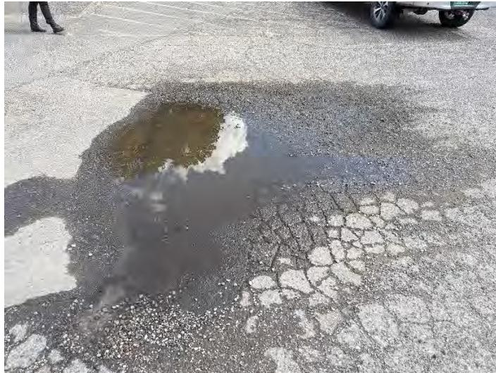
**Picture 1, Pavement failure near northern area inlet**
