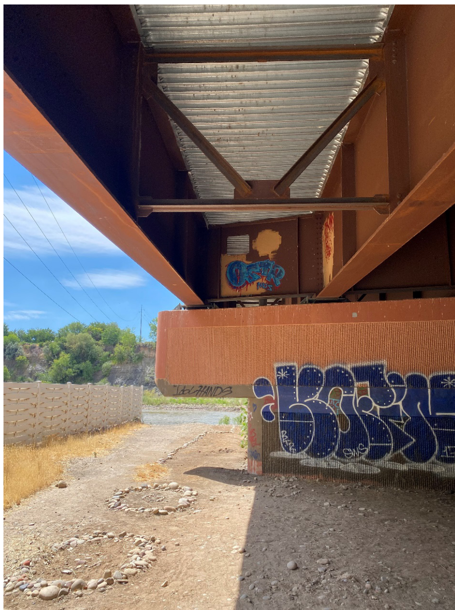
Figure 6 Utility Window in Existing 29 Rd Bridge
