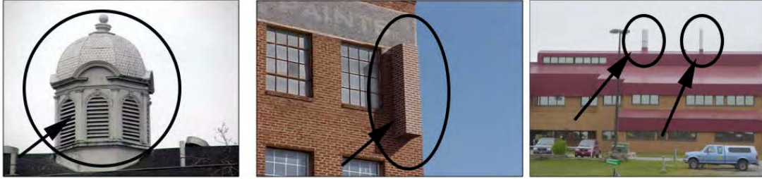
Figure 6: Examples of Antenna Concealment Techniques
