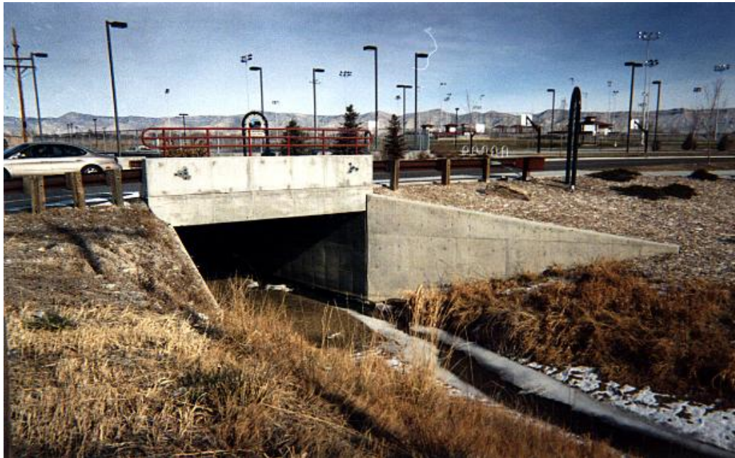
Leach Creek drainage structure near Canyon View Park
