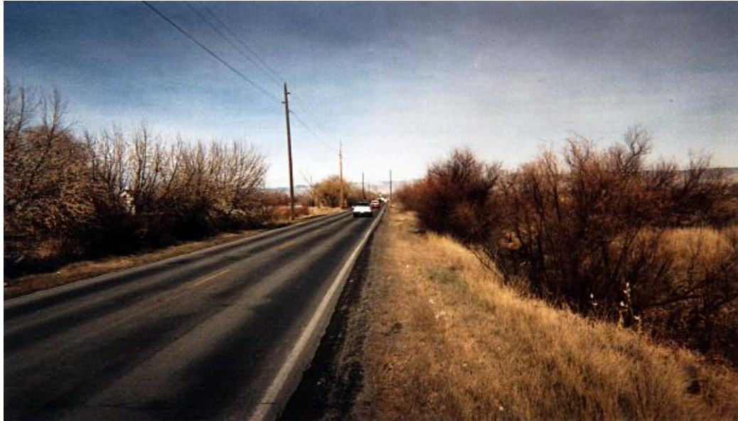
Existing conditions along 24 Road, including Leach Creek on the right
