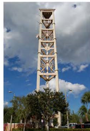
Modified Lattice Tower
