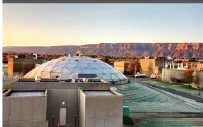
Persigo Wastewater Treatment Facility
