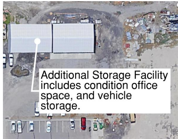
Figure 7.8 Additional Storage Facility
