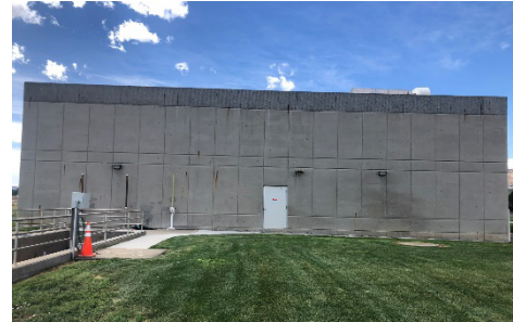
Headworks Building exterior.
