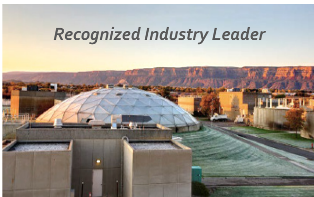
Persigo Wastewater Treatment Facility
