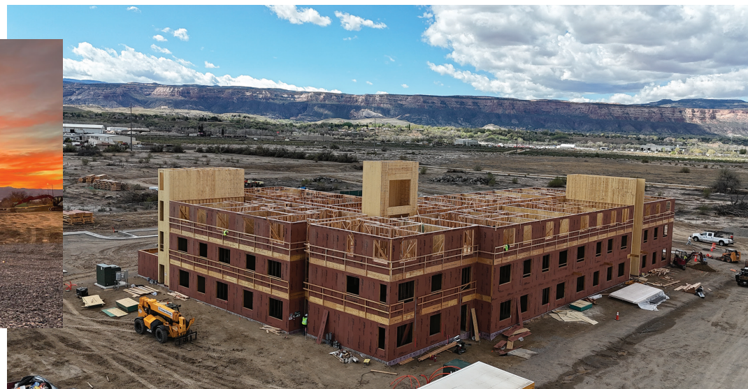
Third floor framing taken April 2, 2026
