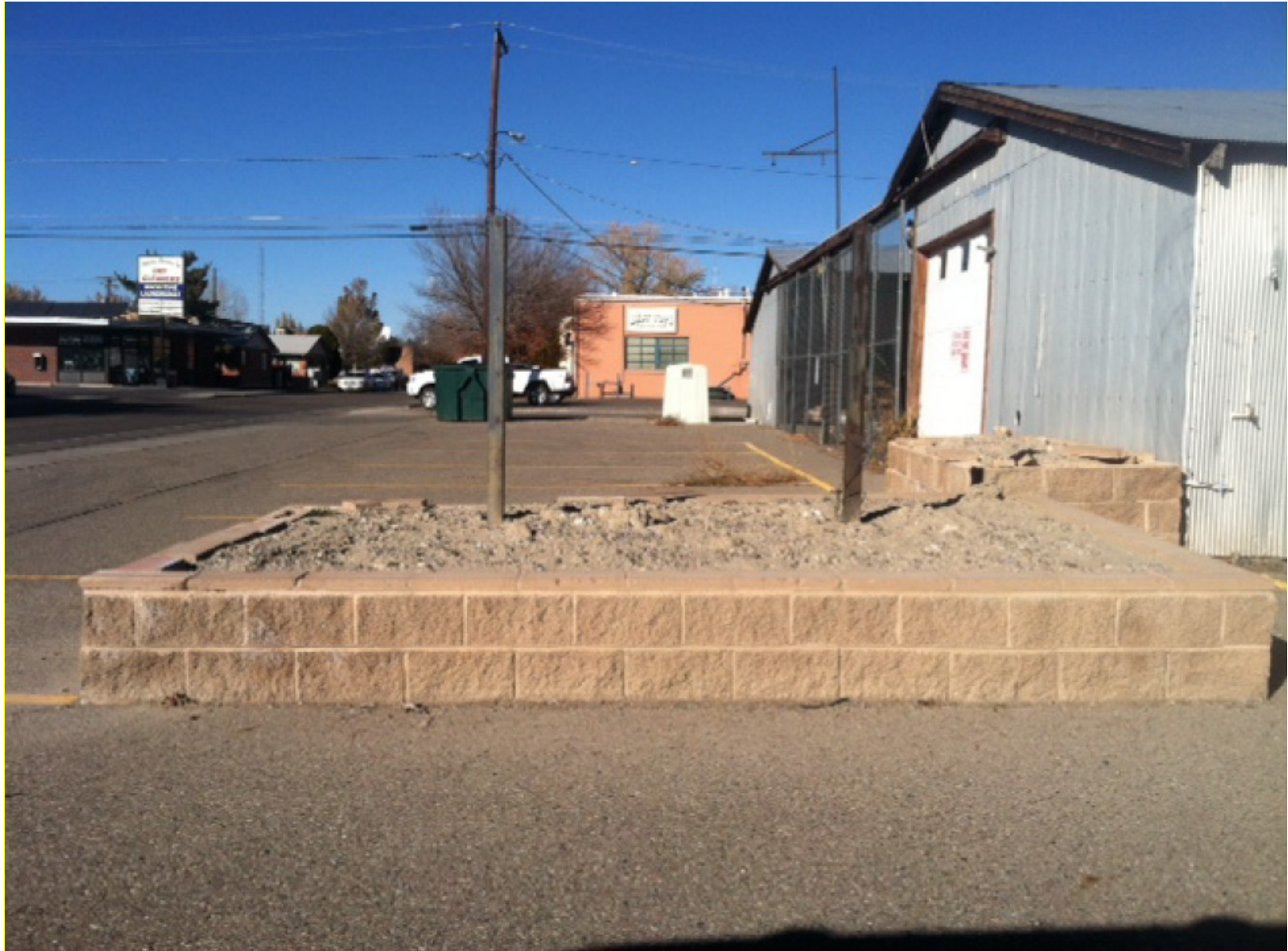
EXISTING SIGN POSTS
