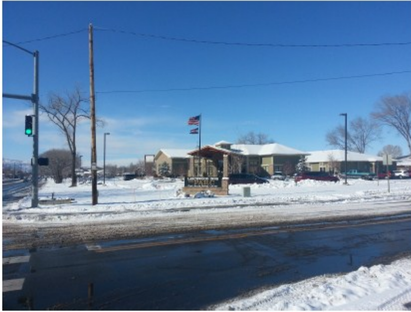
Figure 4. photos of nursing facilities on NW and SE corners
