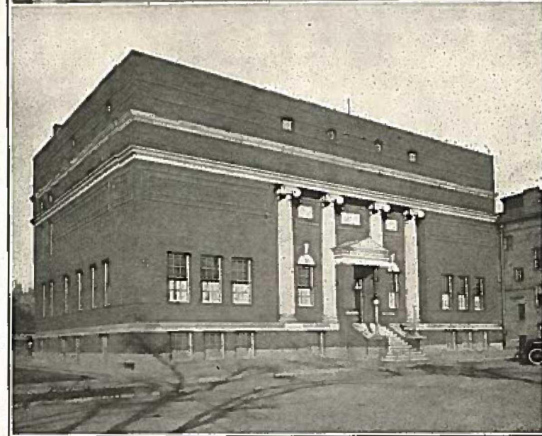
UPPER—FEDERAL BUILDING LOWER—NEW MASONIC TEMPLE—Constructed In 1922
