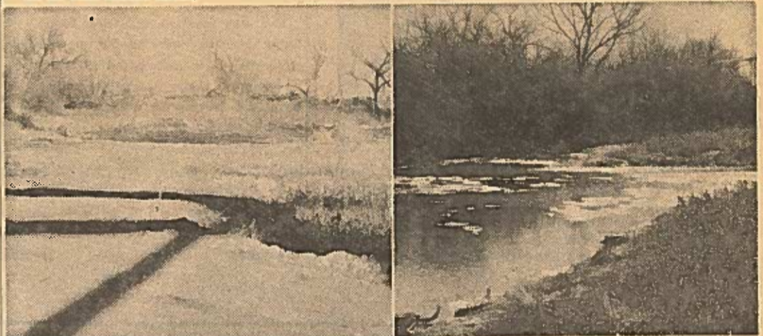
The City's new landfill area is eliminating stagnant ponds of water near the Colorado River (left above). Each night the daily refuse collection is covered with dirt as land is reclaimed for industrial usage as shown right above. The operation has been cited by the County and State Health Departments as one of the most needed sanitation improvements in the area. Only City packer trucks are permitted to dump in the tightly controlled land reclamation project.
