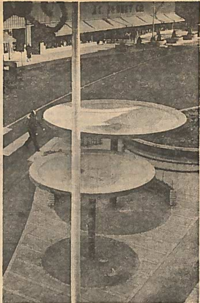
Four concrete canopies in each Shopping Park block provide shade for benches underneath. Public telephones and ground lighting are also featured.
