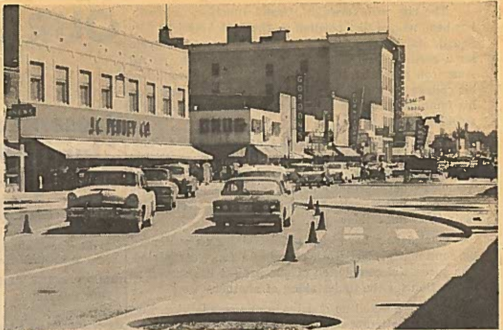
The gentle S-curved lanes of the Shopping Park are part of the design which makes the new concept safer for traffic. During the 1962 Christmas shopping there was only one traffic accident on Main Street compared to six during the same period a year earlier.
