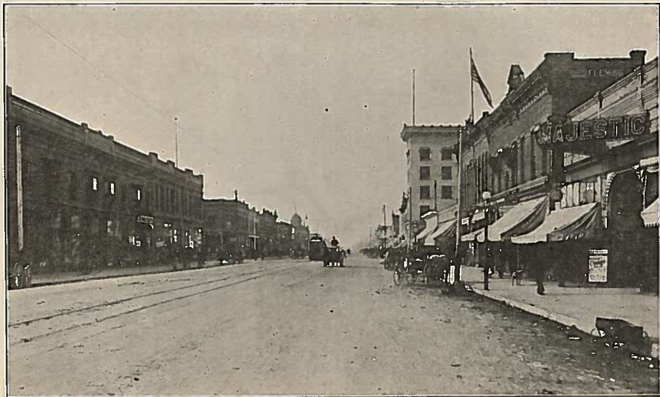
Looking West on Main Street
