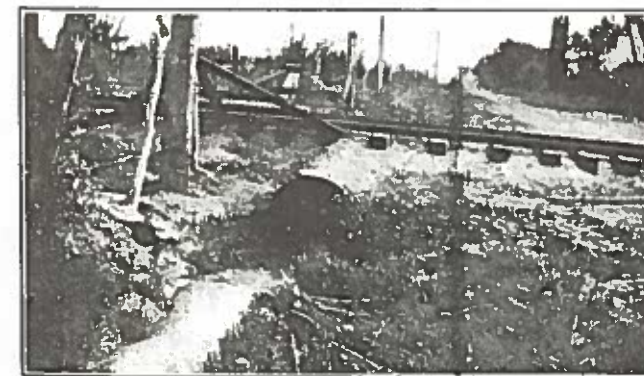
Grand Junction & Grand River Valley Railway—One of the Corrugated Culverts
