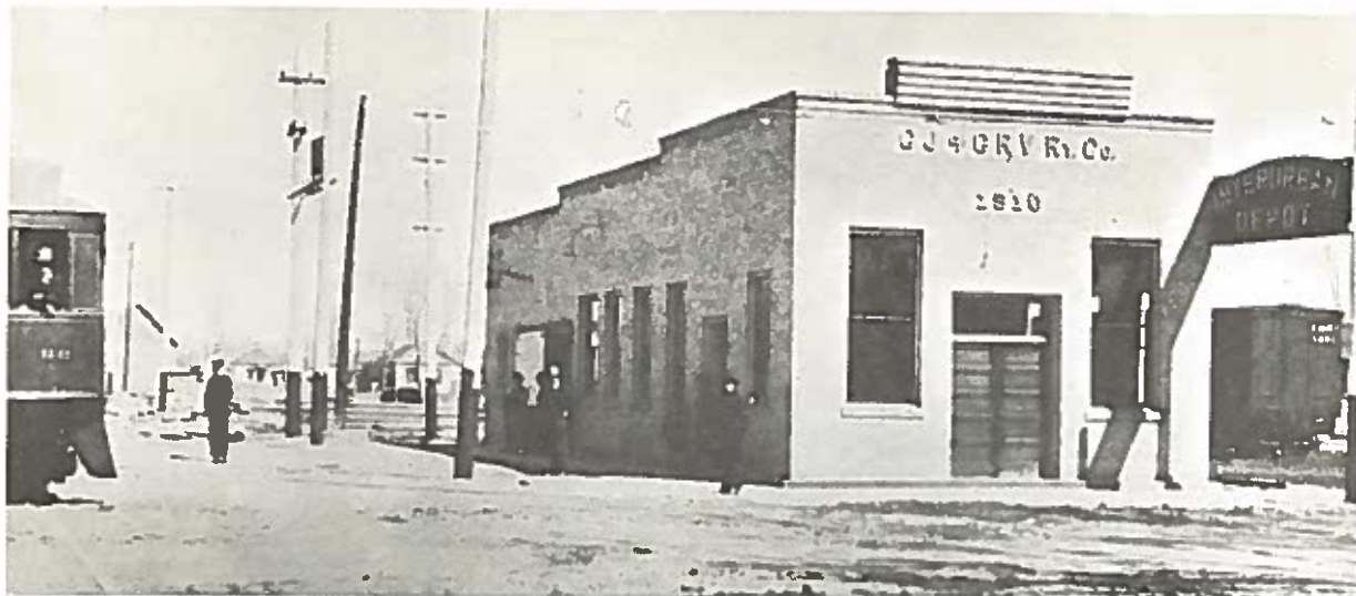
YELLOW BRICK made a neat little depot for Fruita. An electrical sub-station was in the back, dropping the high transmission voltage to the 600 volts D.C. for the cars.
