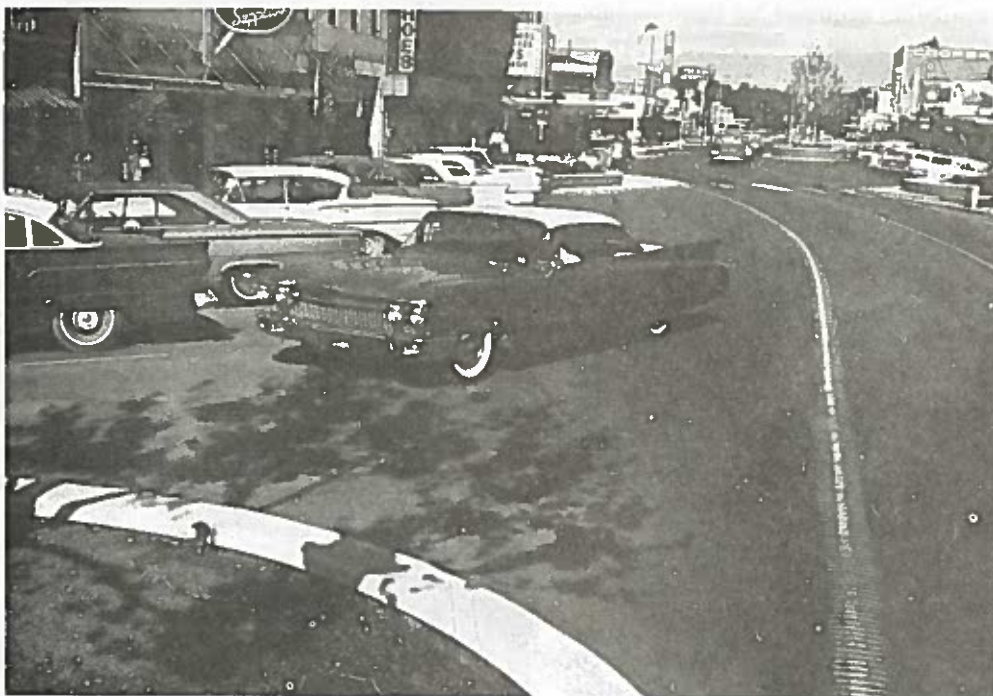
Parked cars have the benefit of a ten-foot-wide maneuvering area so that they do not interfere with moving traffic; note the corrugated concrete "hummer strip" that warns motorists to keep in their travel lanes.
