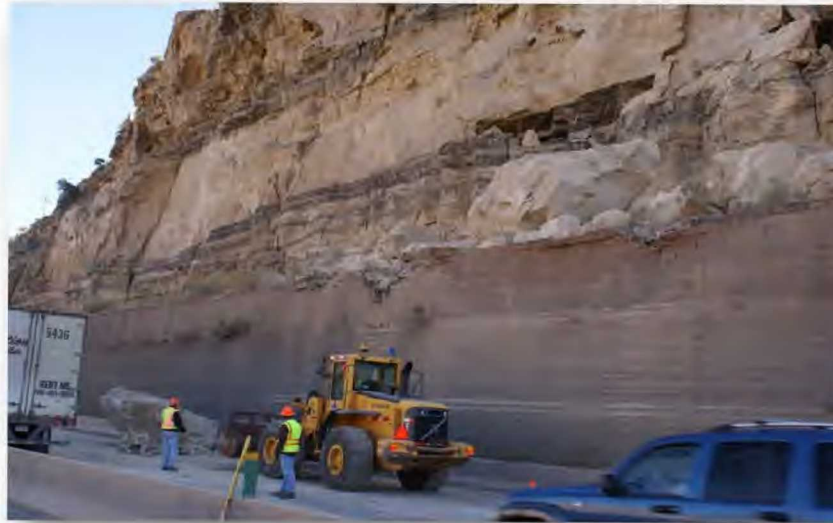
FIGURE 14 ROCKFALL EVENT IN DEBEQUE CANYON AT BEAVER TAIL TUNNEL ON INTERSTATE 70
