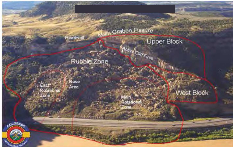
FIGURE 10 DeBeque Canyon Slide Area
