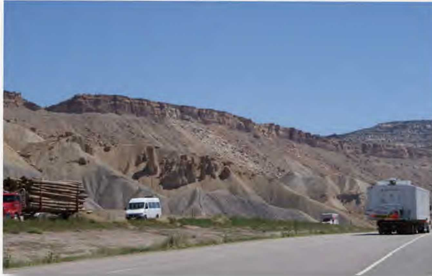
FIGURE 13 ROCKFALL WEST OF PALISADE ALONG INTERSTATE 70
