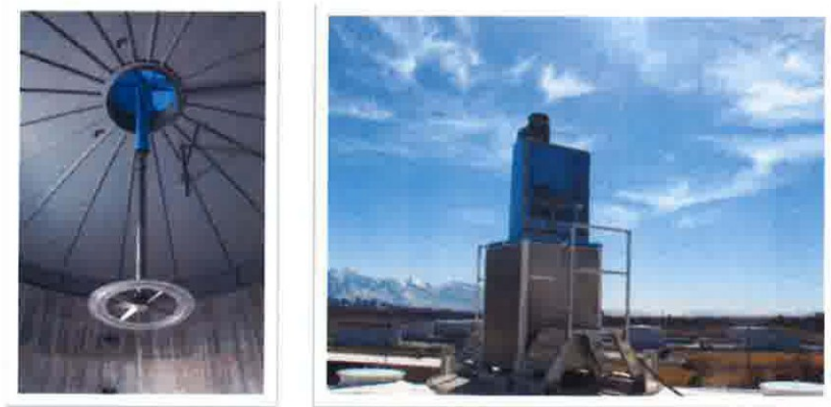
Figure2: LM™ Mixer (showing both inside of tank and top of cover)
