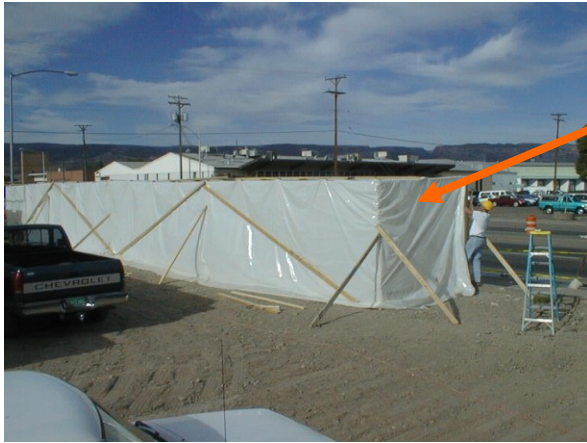
Tent covering for asbestos removal
