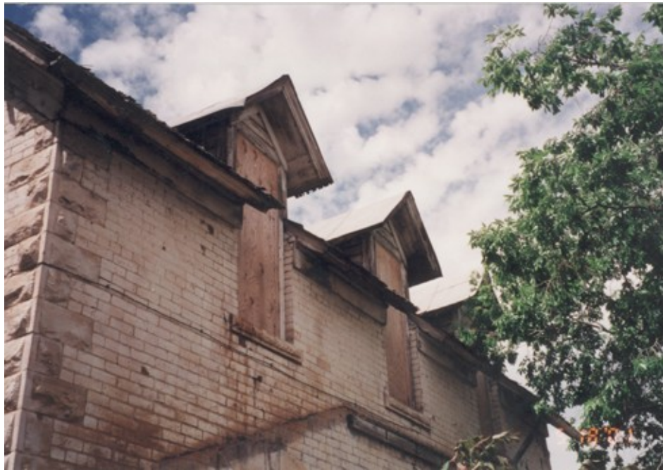
6. The north face bedroom gabled dormers.
