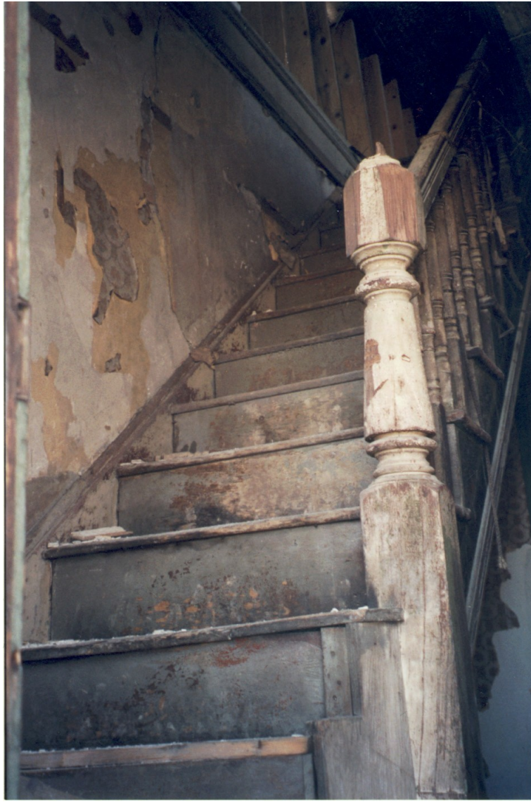
31. View of the stairway to the second floor level.
