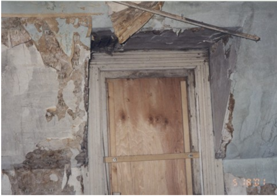
25. Interior northwest second story bedroom dormer from inside.
