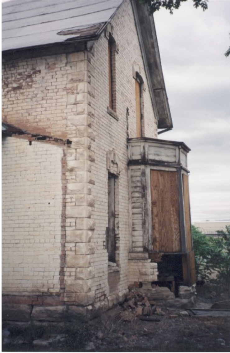
17. East side of two story portion at the damaged and boarded up bay window. Also shown is outline of east porch that has been demolished.
