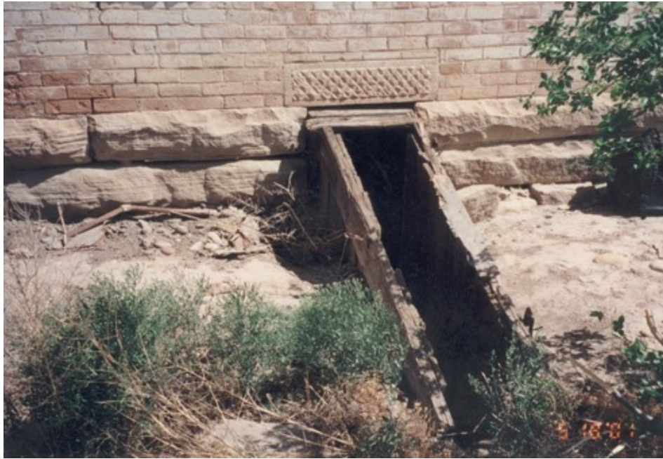
13. Basement access with on south side with ornamental sandstone lintel.
