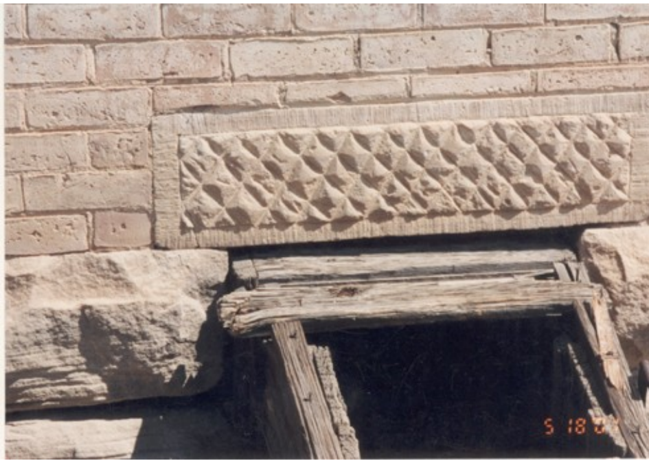
14. Crisscrossed sandstone lintel at basement entrance and wood framed entry.
