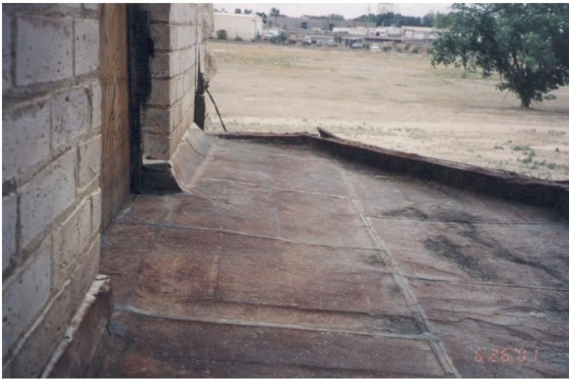
19. Top of east side bay window – boarded up door opening leads to upstairs master bedroom
