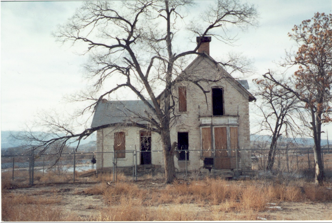
3. East side showing bay window.
