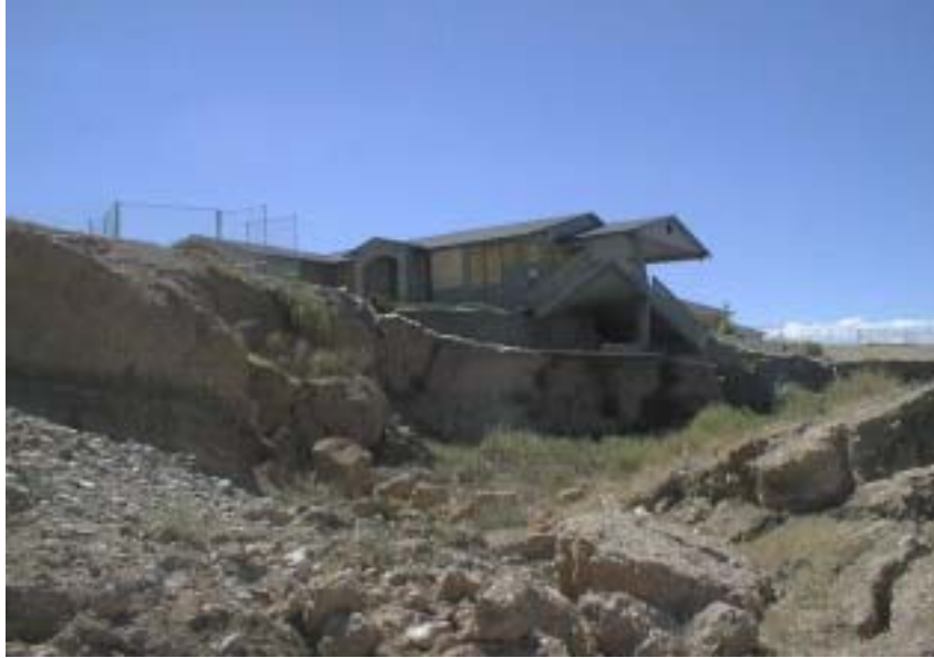
Unstable Slopes along the bluffs south of the Colorado River, west of the Redlands Parkway
