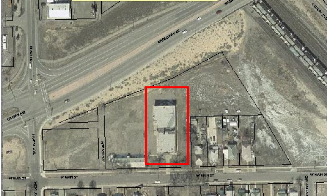
CDBG 2004-08(a) RIVERSIDE SCHOOL ROOF REPAIR 552 WEST MAIN STREET
