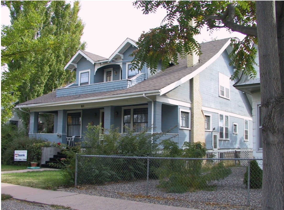
CDBG 2004-11 HOPE HAVEN ROOF REPLACEMENT
