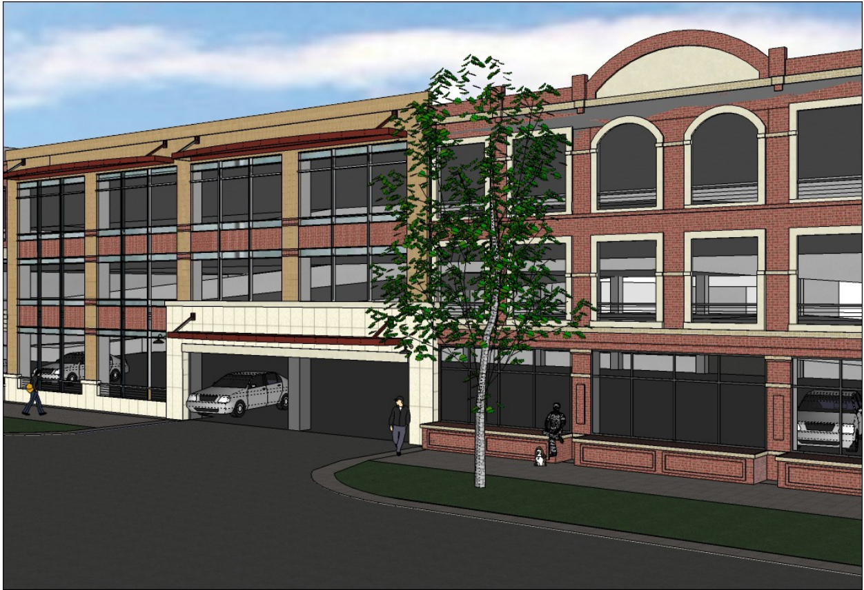
East End of the Garage
