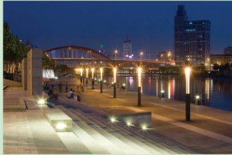
Haihe River Embankment - Tianjin, China
