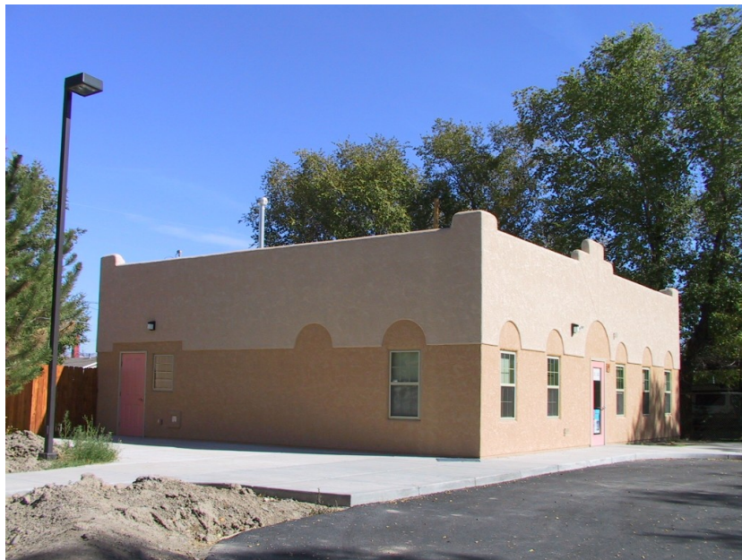
Existing Head Start Facility to be Expanded Constructed 2002 with CDBG Funds
