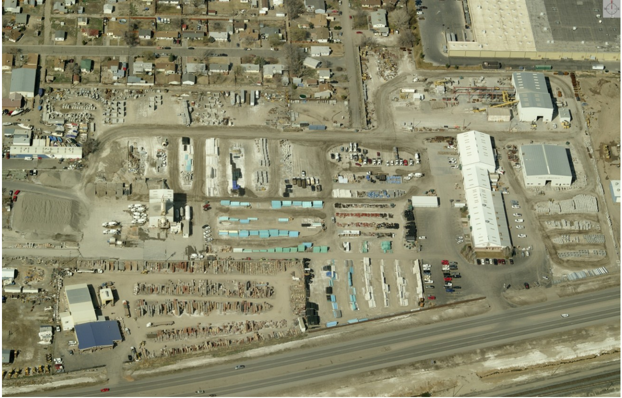
Grand Junction Pipe / Non Conforming site
