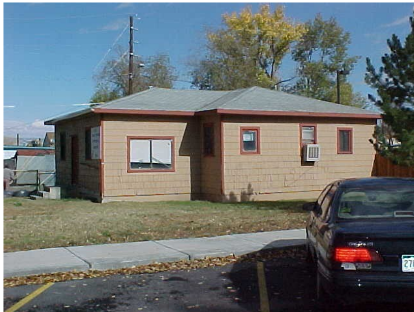
Existing Vacant/Storage Structure Potentially Remodeled for Additional Classroom
