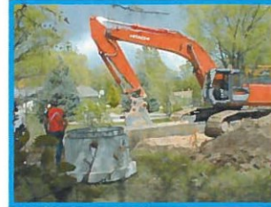
Skyway Sewer ID
