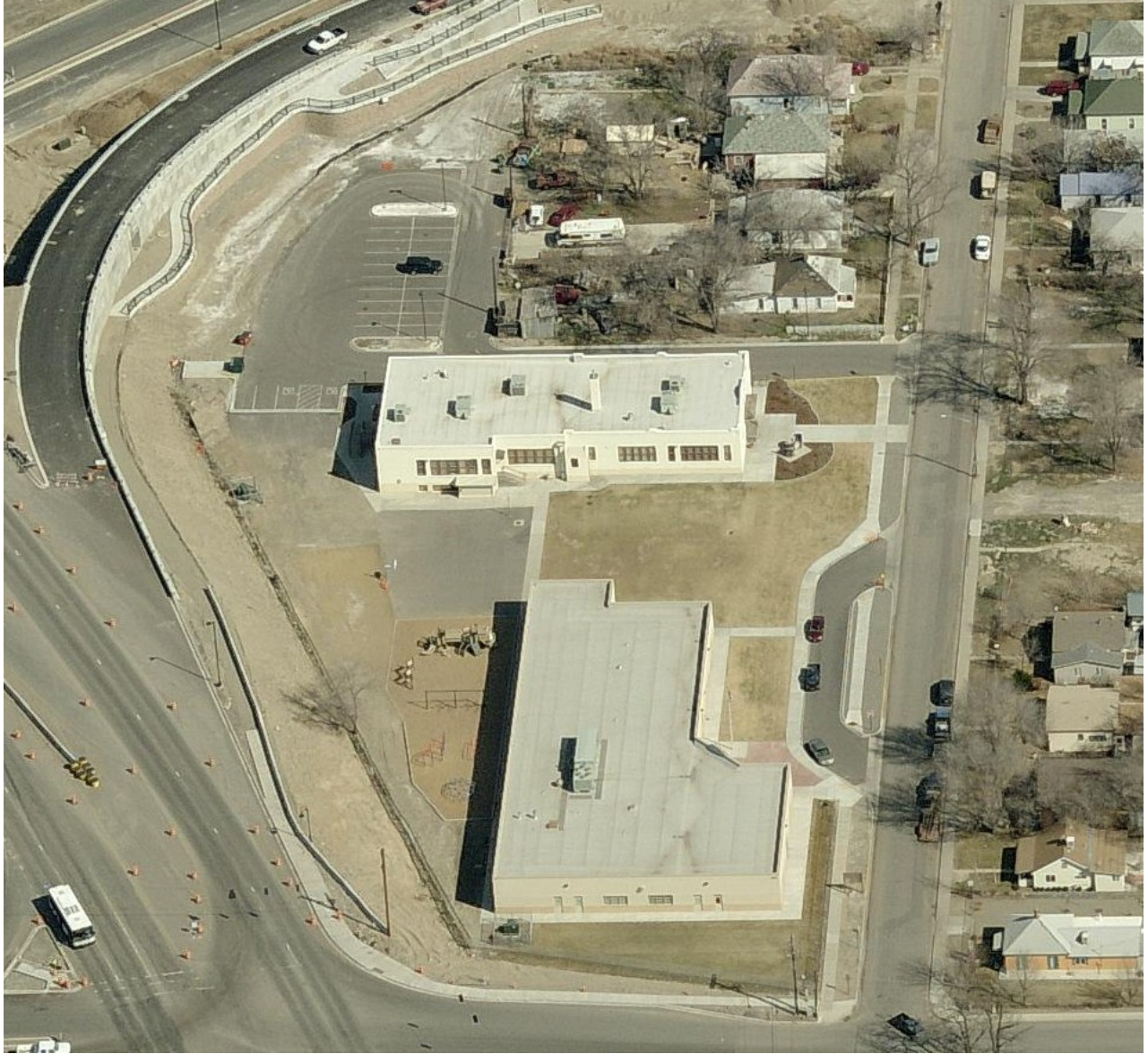
CDBG 2009-09 DUAL IMMERSION ACADEMY SLOPE STABILIZATION AND LANDSCAPING
