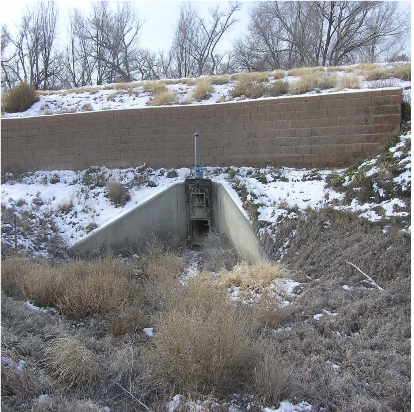
5) Outfall structure located at the southwest corner of the project.
