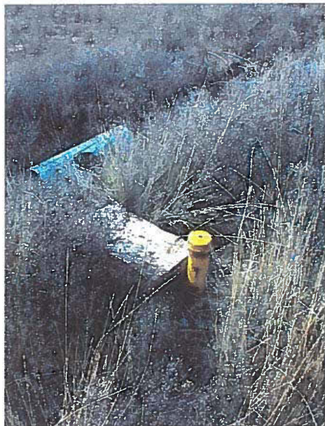
Standpipe Near Northeast Corner of Subject Property
