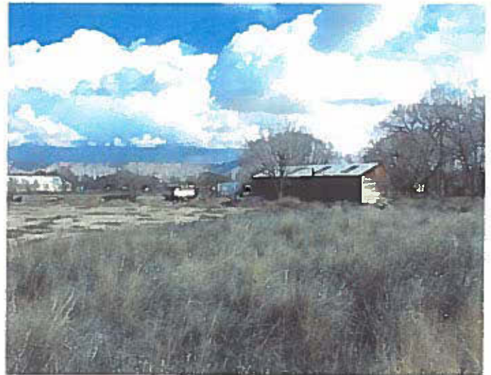
View Northeast of Garage/Shop Building
