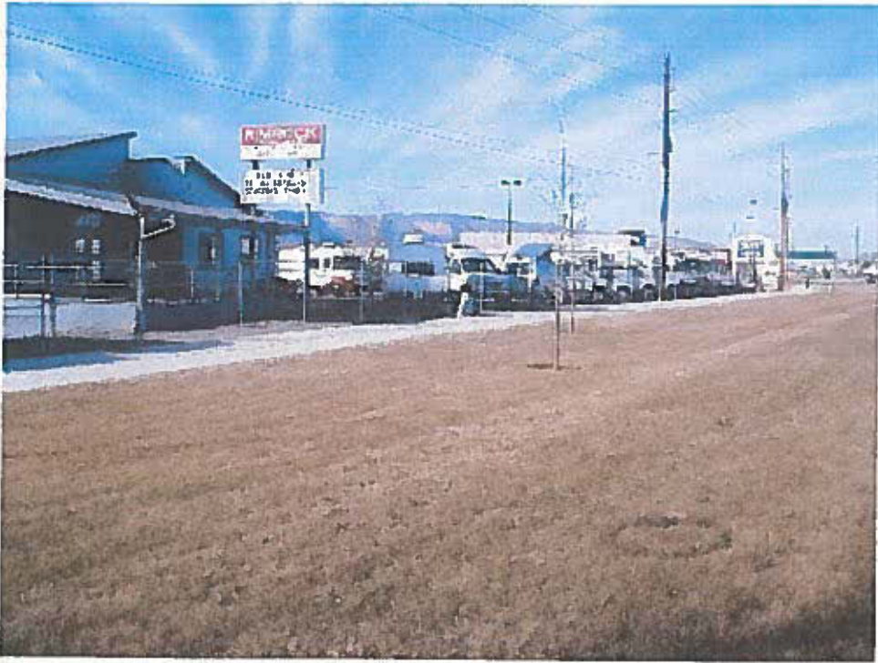
5. Standing adjacent to Highway 6&50 looking southwest at existing building and property.
