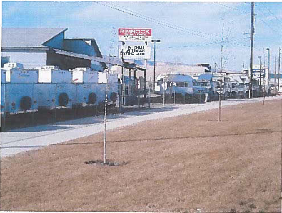
7. Standing adjacent to Highway 6&50 looking southwest at existing building and property.
