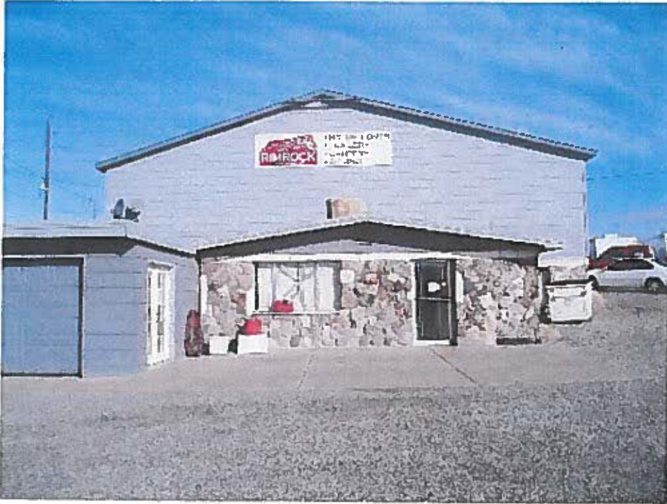
1. Standing in the parking lot looking north at the existing building.
