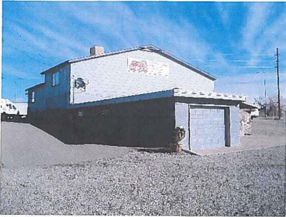
3. Standing in the parking lot looking northeast at existing building.
