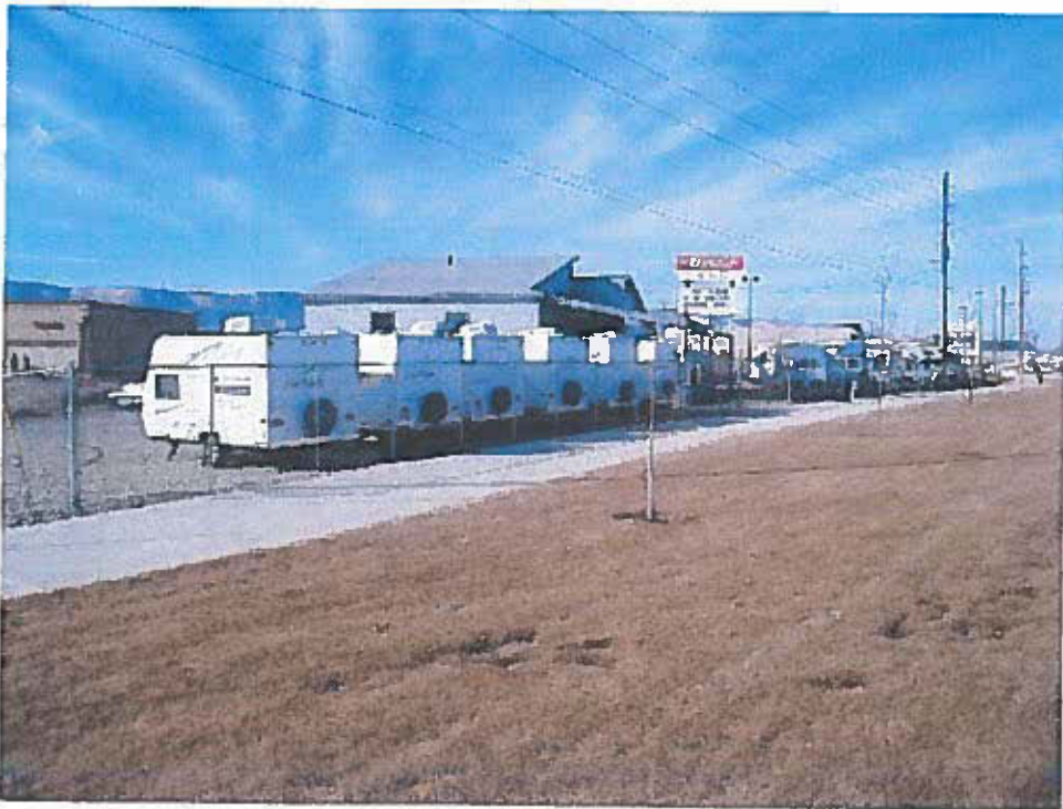
6. Standing adjacent to Highway 6&50 looking southwest at existing building and property.
