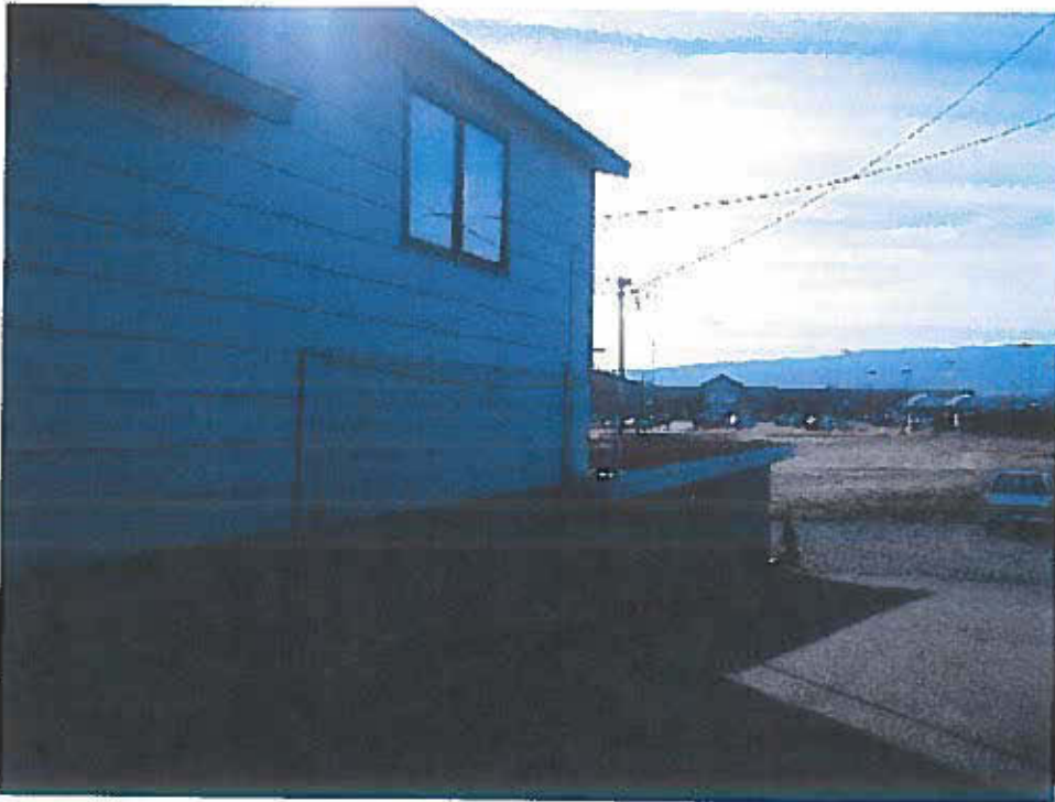
4. Standing in the existing parking lot looking south at existing building. Note Wal-Mart Facility in background.
