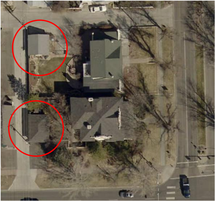
Typical Scale of Historic Accessory Structures in the North Seventh Street Historic Residential District
