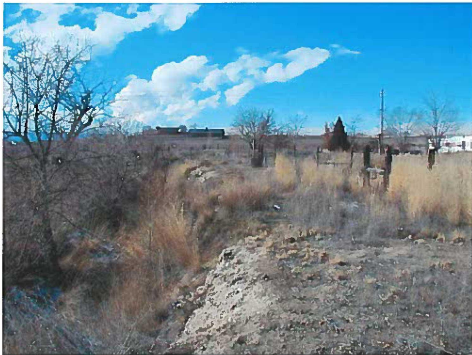
Photograph 4 – Irrigation Canal. View to the west.
