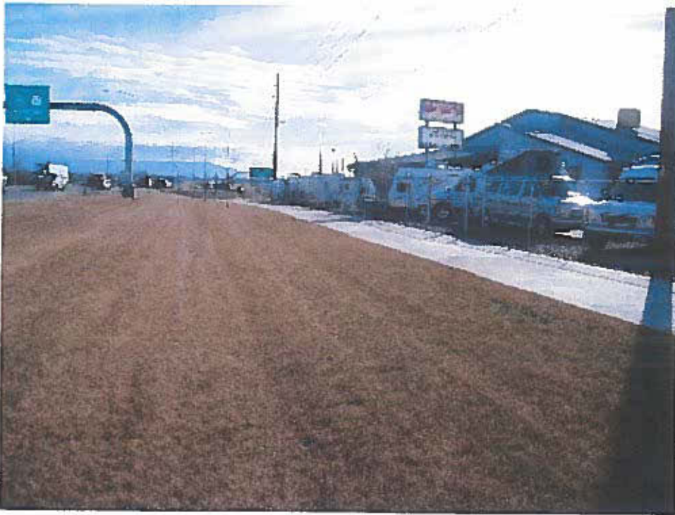
12. Standing adjacent to Highway 6&50 looking east at existing building and property.
