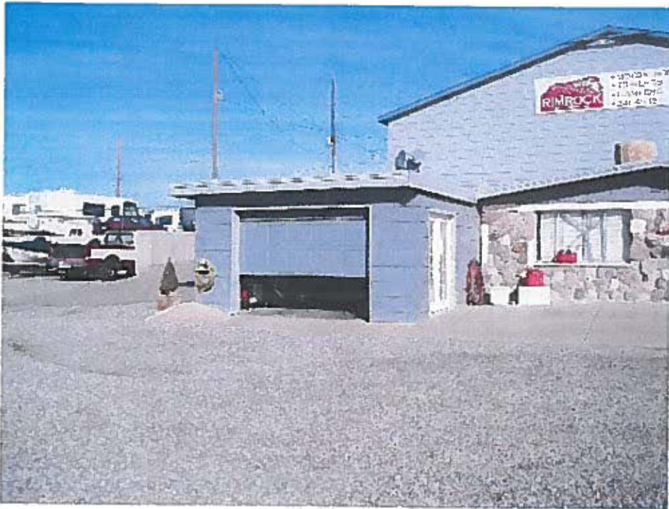
2. Standing in the parking lot looking northwest at existing building.
