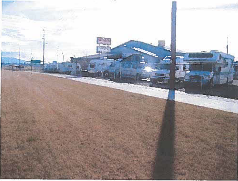
11. Standing adjacent to Highway 6&50 looking east at existing building and property.
