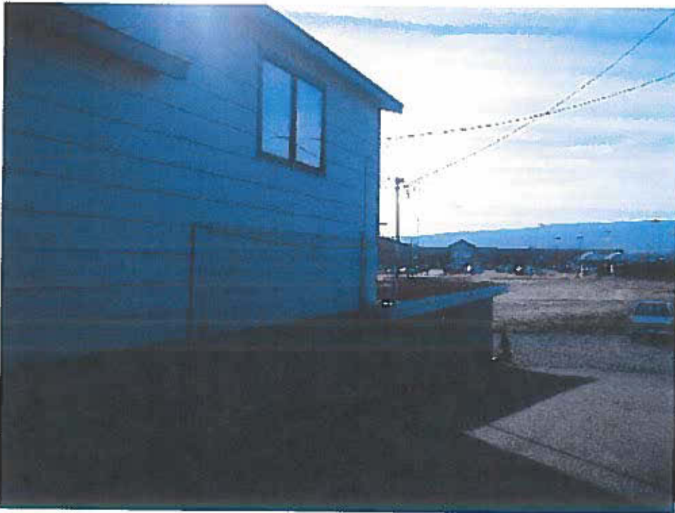
4. Standing in the existing parking lot looking south at existing building. Note Wal-Mart Facility in background.
