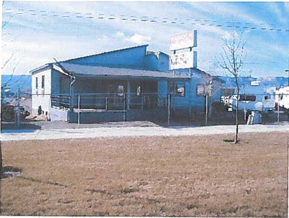
9. Standing adjacent to Highway 6&50 looking south at existing building and property.
