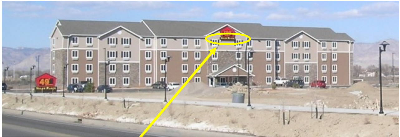
View of Value Place Hotel from 24 Road – 12 inch letters
