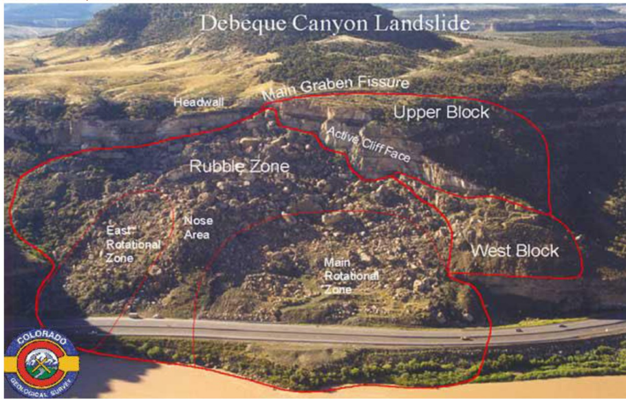
FIGURE 10 DEBEQUE CANYON SLIDE AREA
