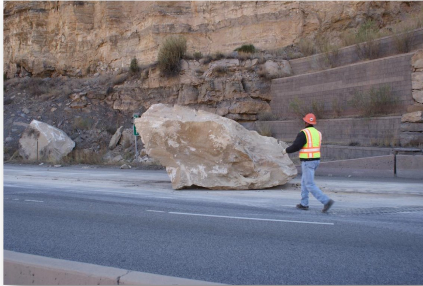
FIGURE 15 ROCKFALL EVENT IN DEBEQUE CANYON AT BEAVER TAIL TUNNEL ON INTERSTATE 70
