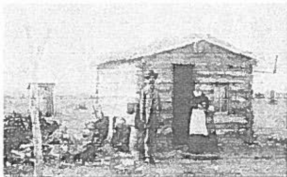
(F-361) Figure 2. The first cabin in Grand Junction was built in 1881, of cottonwood logs with a sod roof. It was located at the intersection of Ute Avenue and 2nd Street.
