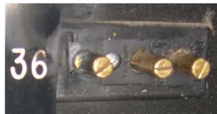
Short in Inlet Panel Circuit #36 Connector
