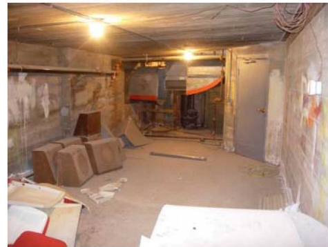
Under Stage Basement
