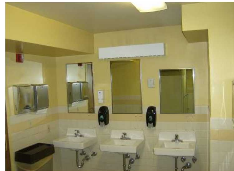
Typical Existing Lavatories
