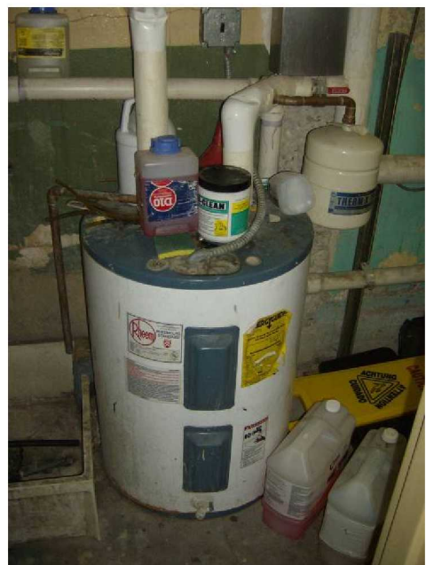
Typical Electric Water Heater
