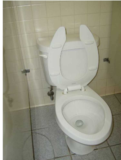
Typical Existing Water Closet
