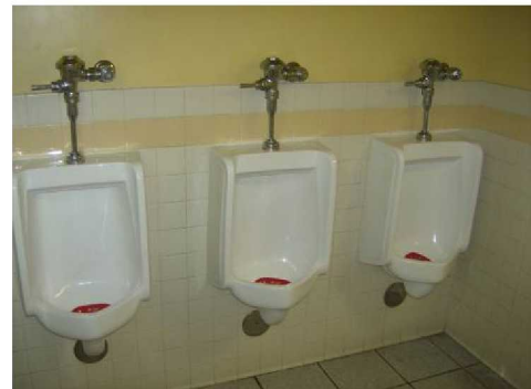
Typical Existing Urinals
