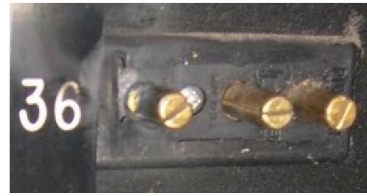
Short in Inlet Panel Circuit #36 Connector
