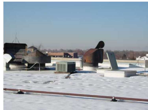
Roof and Roof mounted equipment
