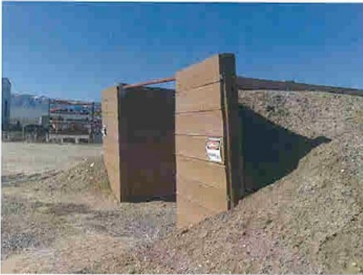
Photos of example storage bunker
