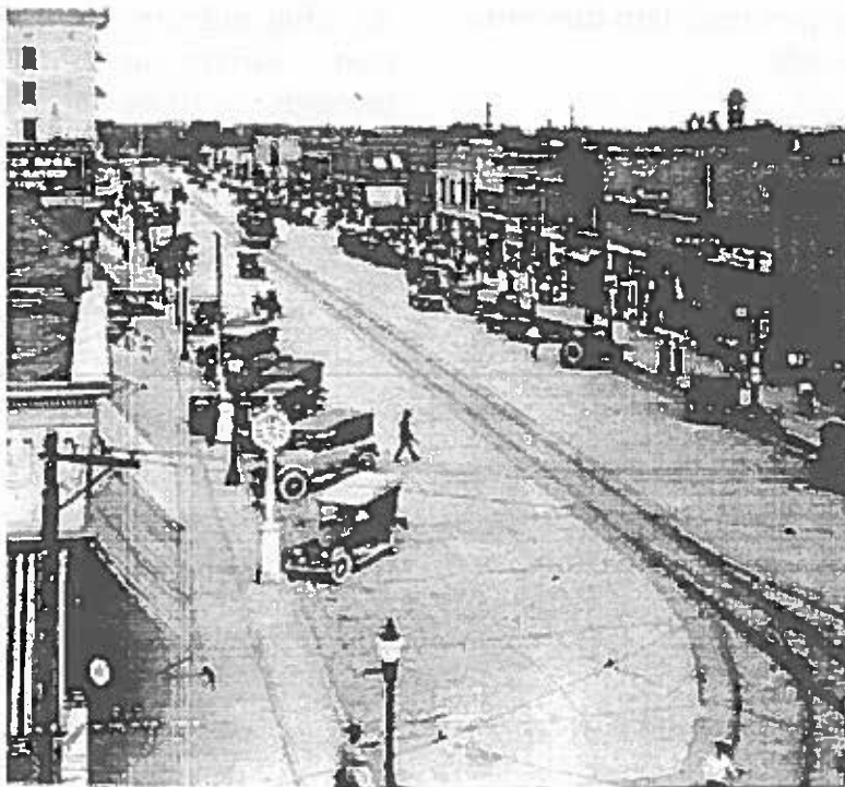
Downtown in 1917 had paved streets with street car rails and acorn-style street lights. (Photo: Courtesy of Museum of Western Colorado)
