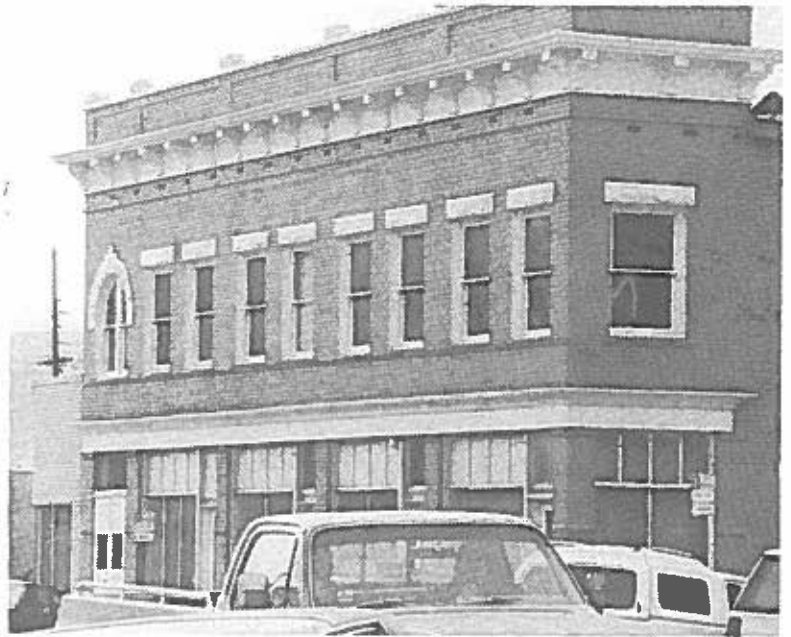
Several downtown buildings survive with a high degree of architectural integrity.
