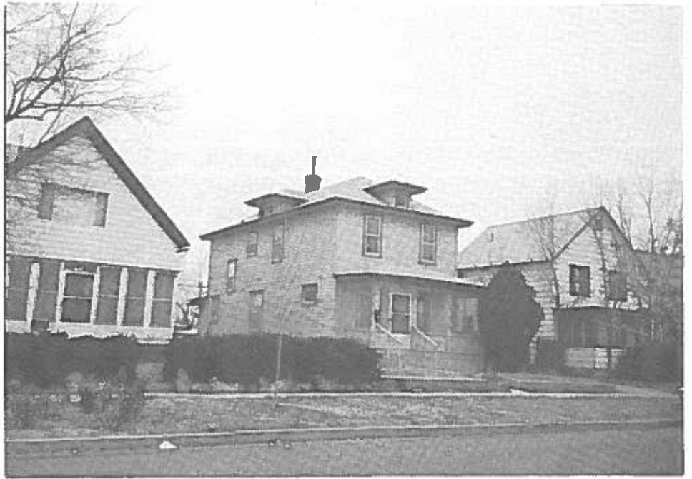
Site plans and landscape materials may also contribute to the character of some neighborhoods.
