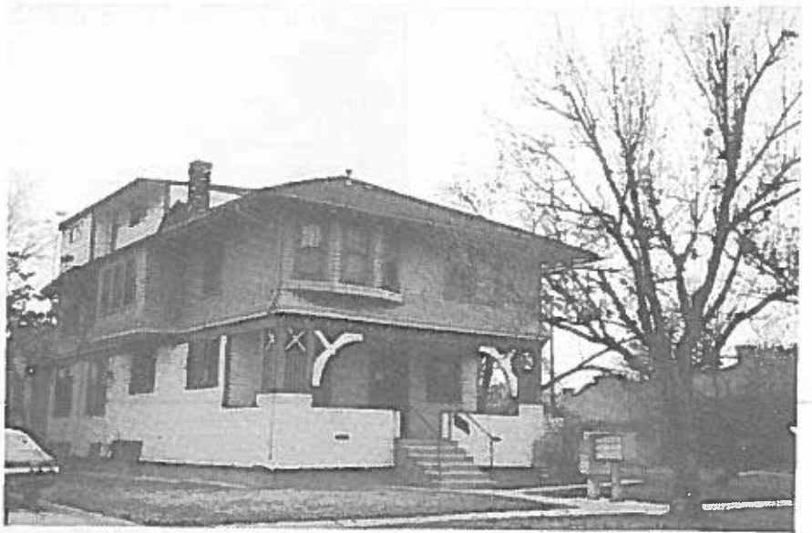
This multi-family structure exhibits craftsma style details, including sculpted shingled walls and exposed eave brackets. Later alterations have slightly affected its character.
