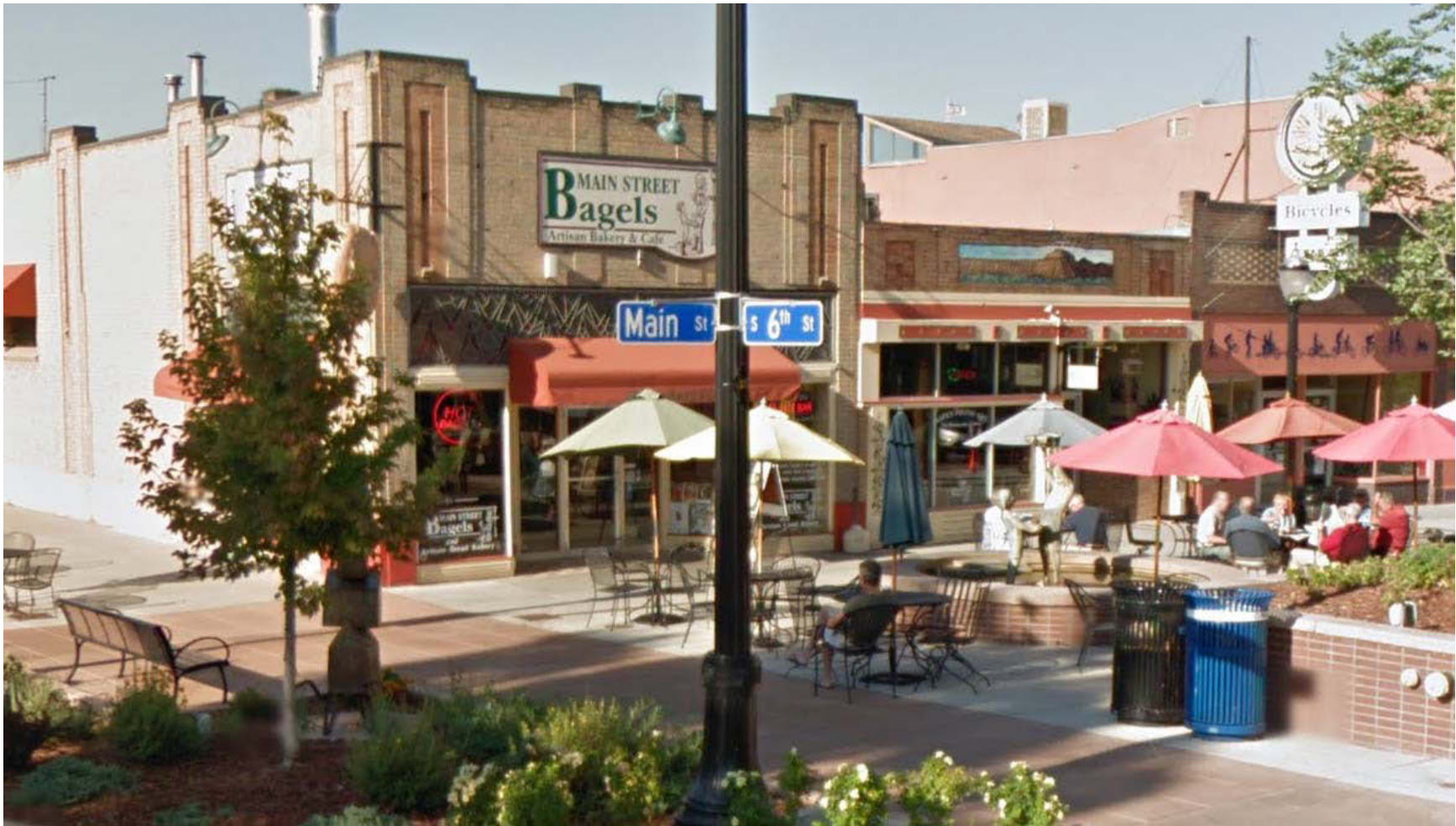
559 Main Street Current Google Street View July 2012
